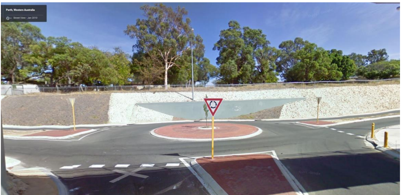
Existing Site Conditions- view looking northwest towards site with retaining wall and embankment at Nagal Pass/Stubbs Terrace
