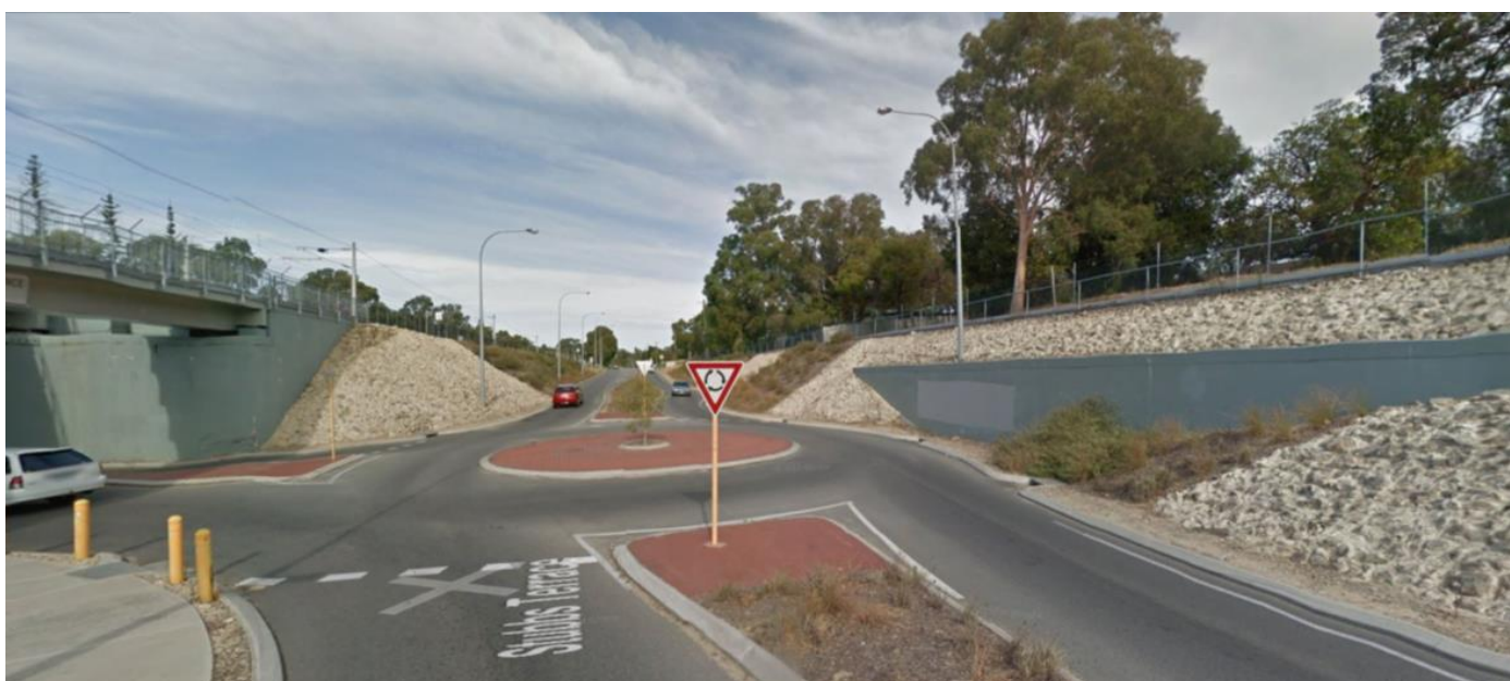
Existing Site Conditions- view looking southwest towards site with retaining wall and embankment at Nagal Pass/Stubbs Terrace Traffic
