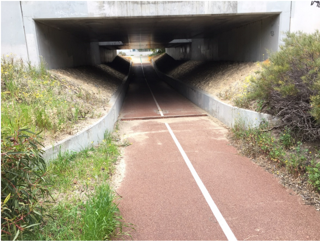
Image 1 (above): underpass approach from Swanbourne side
