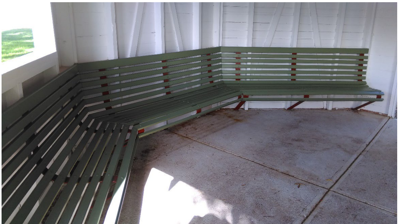
Figure 2: Internal refurbishment - April 2018
