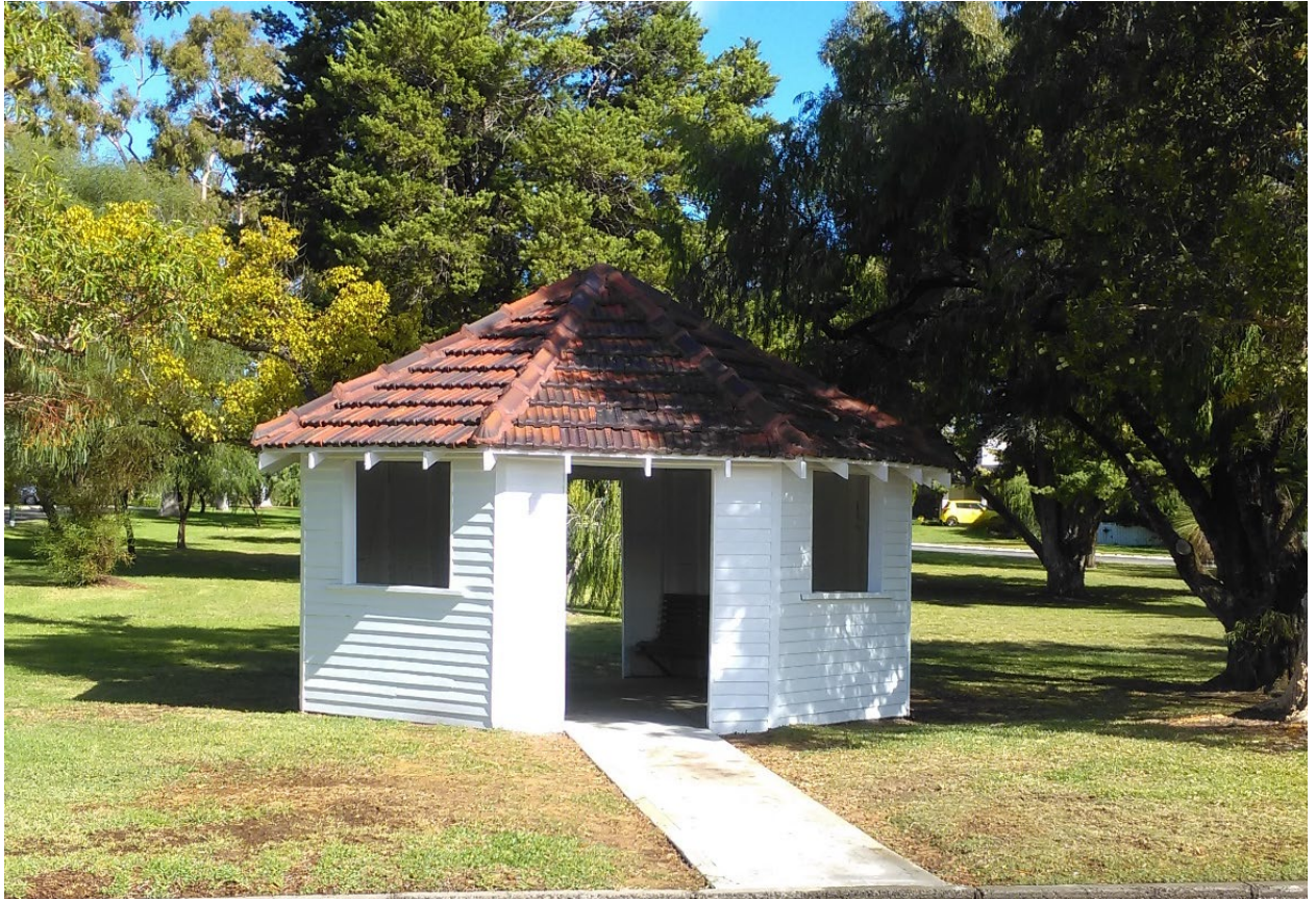
Figure 3: External refurbishment - April 2018
