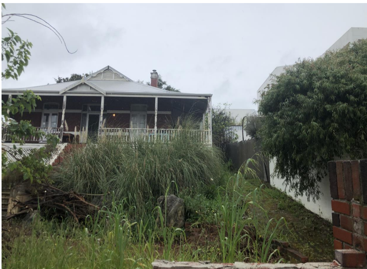
Photograph 4: View of southern adjoining property, facing west from Broadway
