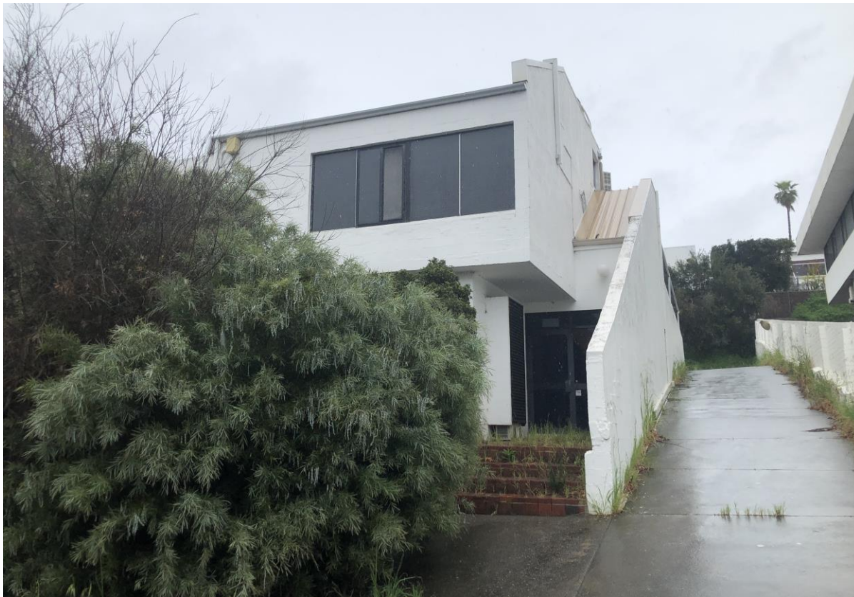
Photograph 1: View of subject site facing south-west from Broadway
