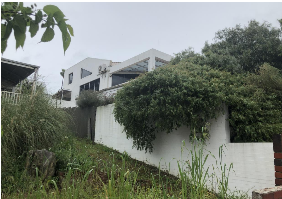
Photograph 2: View of subject site facing north-west from Broadway
