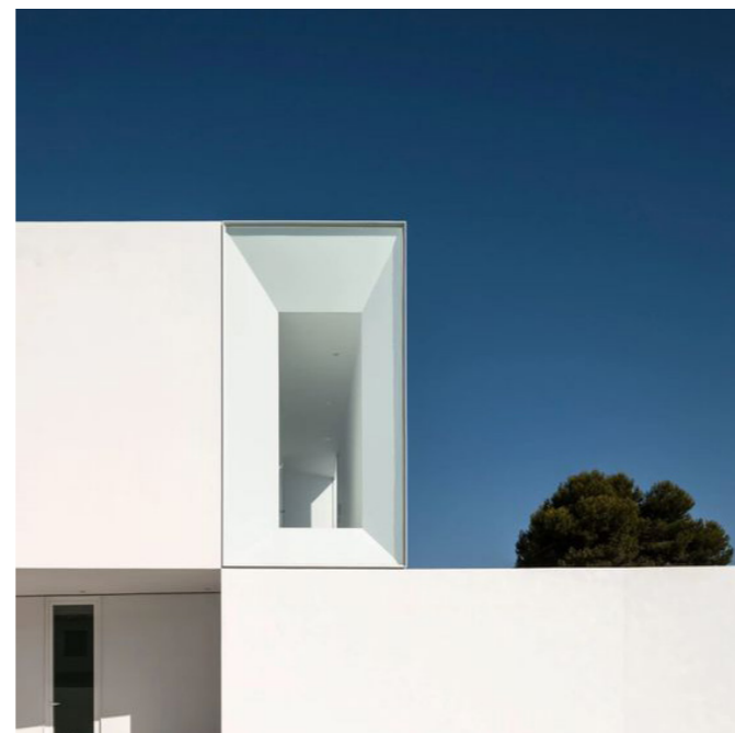
4. Deep geometric building forms play on light and shadow and help break up the elevation of the building. These forms create interest from the street.
