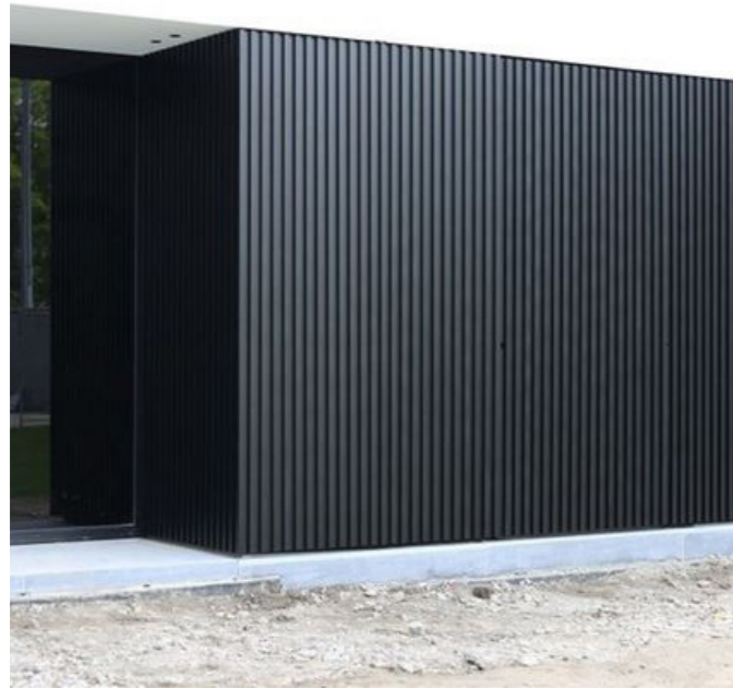
6. Aluminum batten concealed openings minimises the monotonous nature of a length of garage doors across the buildings elevation. This technique also compliments the sleek and contemporary qualities of the development.
