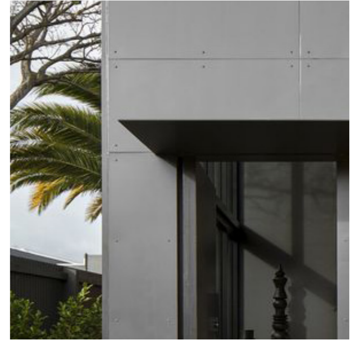
3. Thin awning/ hood over north-facing glazing. Ground floor only.
