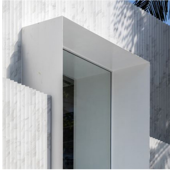
1. Deep steel reveals provide shading and articulation to the building facade.
