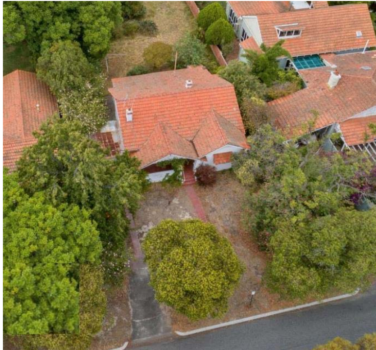
Photograph 1 – Existing land use: Aerial view of existing residence at 24 Clarke St
