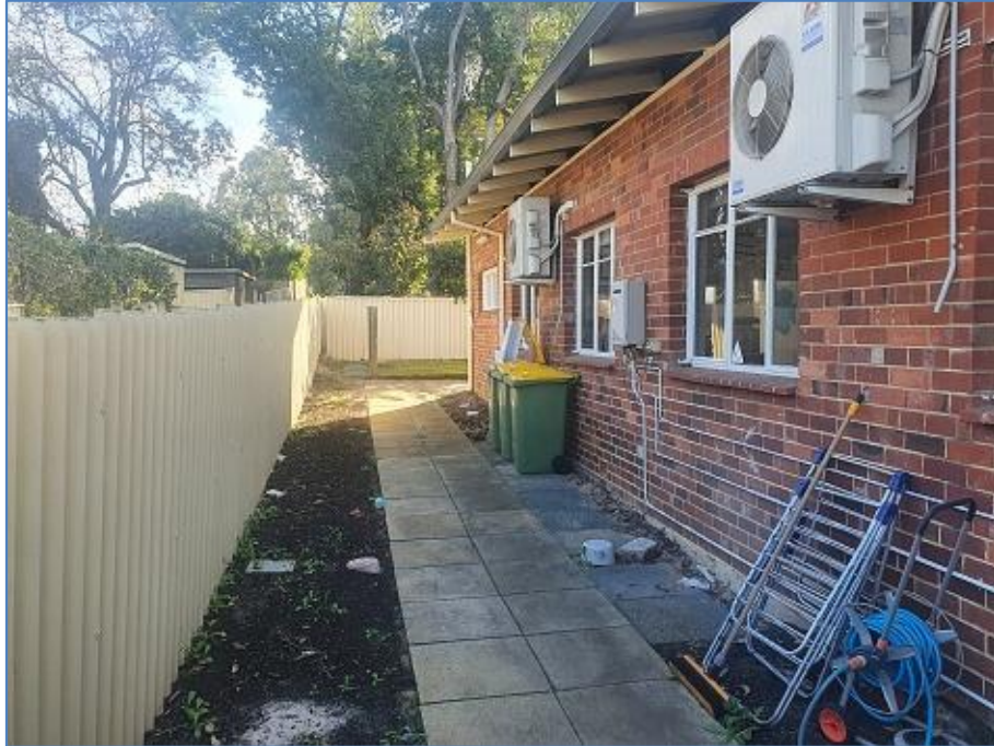
Rear of site
