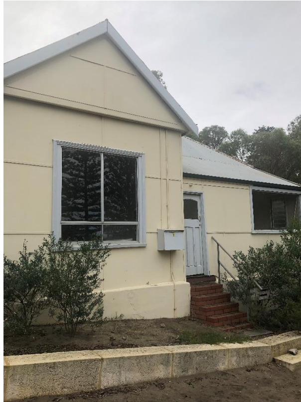
Photograph 1 – Front of Building
