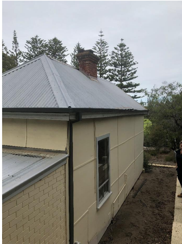
Photograph 5 – West Side of Building-Roof Sheeting Not Fixed Down
