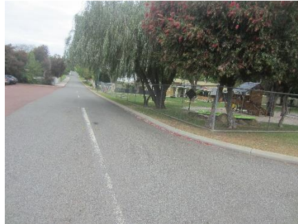
Hackett Road Frontage
