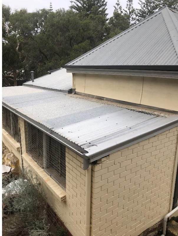
Photograph 2 – Rear of Building
