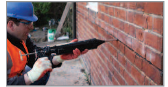
5. Insert a further bead of HeliBond over the exposed HeliBar, finishing 10 – 15mm from the face, and 'iron' firmly into the slot using the HeliBar Finger Trowel
