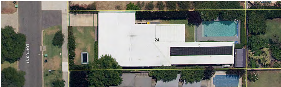
FIG 7. ARIAL PIC OF 24 LOFTUS STREET SHOWING THE EXTENSION THAT EXTENDS WELL OVER ITS BACK SETBACK BOUNDARY.
