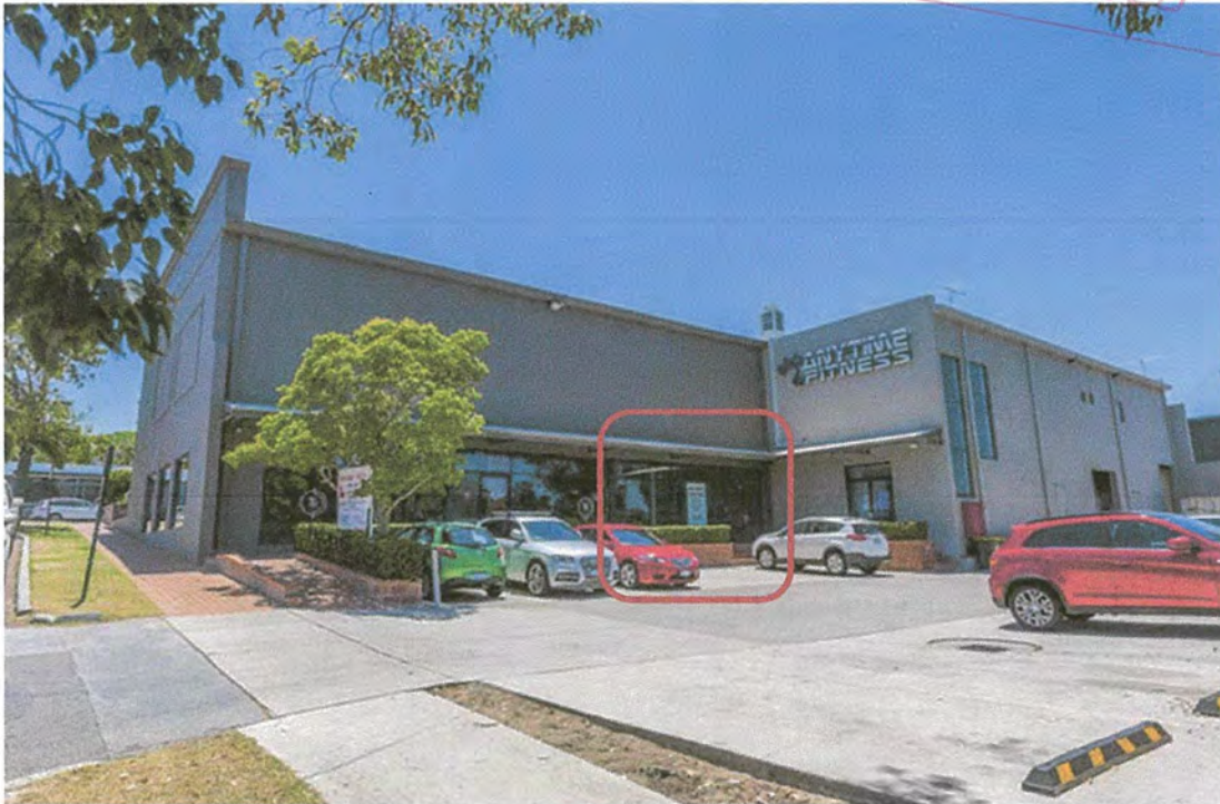
Figure 2 – External photographs of Unit 3A, 150 Stirling Hwy Nedlands
