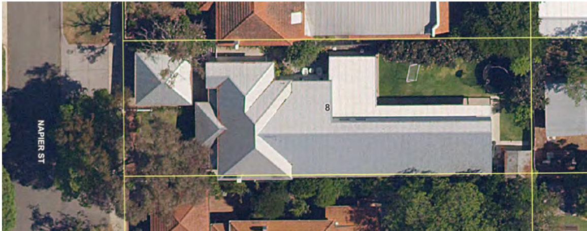
FIG 6. ARIAL PIC OF 8 NAPIER STREET SHOWING THE EXTENSION THAT EXTENDS WELL OVER ITS BACK SETBACK BOUNDARY.
