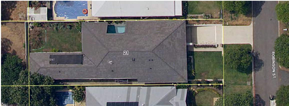
FIG 5. ARIAL PIC OF 21 ROBINSON STREET SHOWING EXTENSION RIGHT TO ITS WESTERN BOUNDARY.
