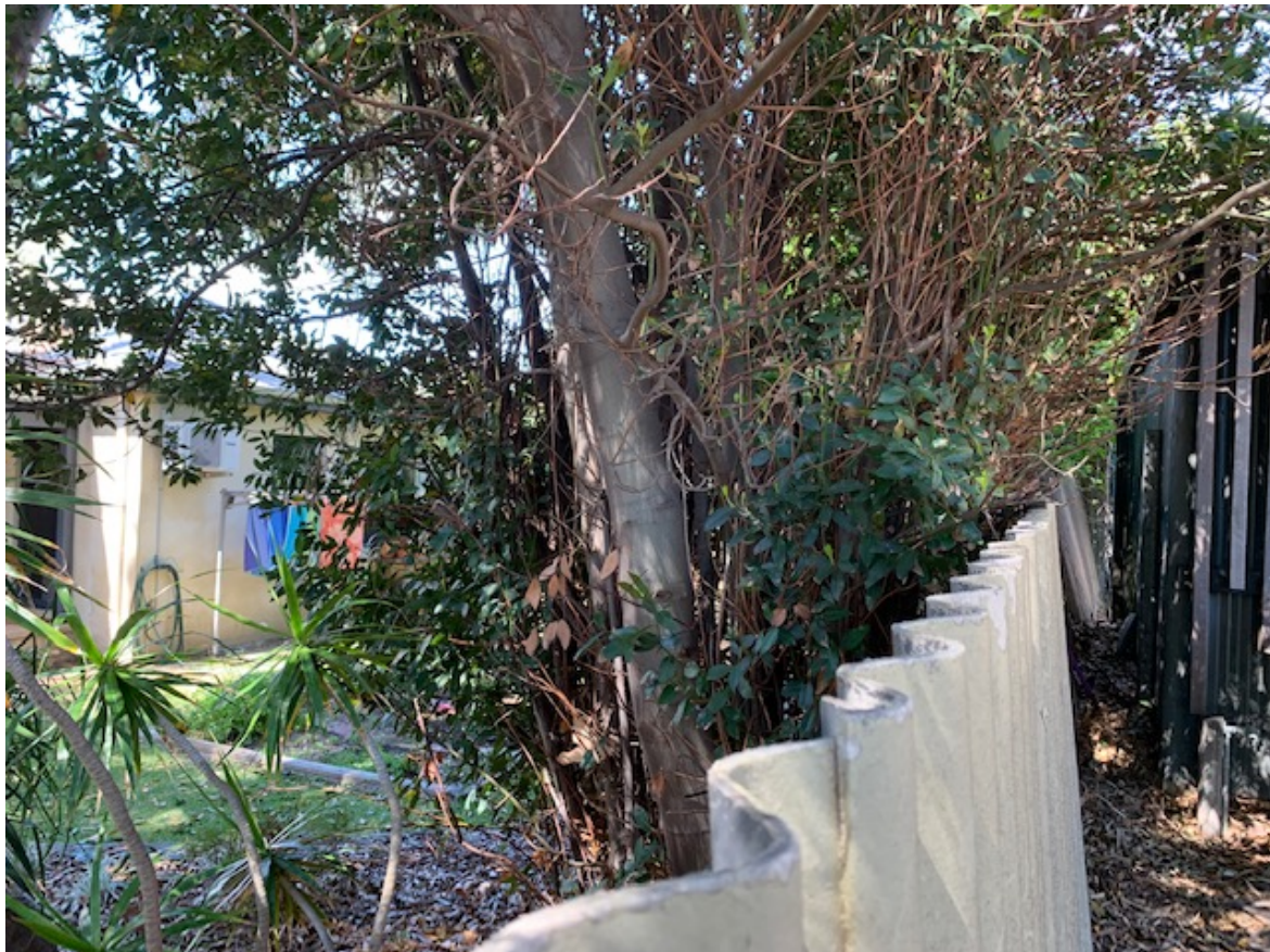
Figure 1: View from street along the existing dividing fence showing the vegetation on the adjoining lot. Proposed garage will be forward of the shed shown on the right.
