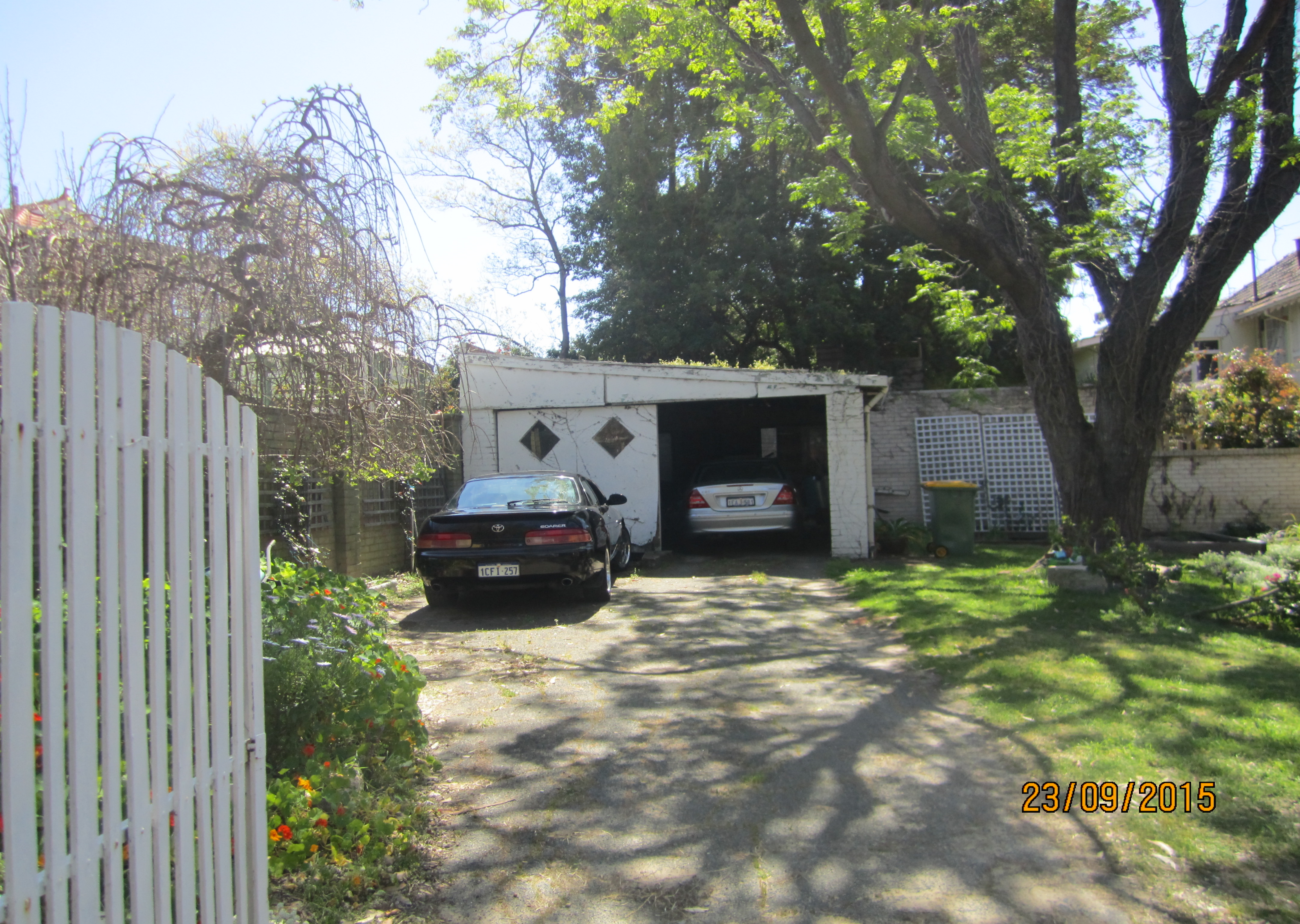
PD52.15 Attachment 4 - Site photograph of 101 Thomas Road as viewed from the secondary street (Melvista Avenue)
