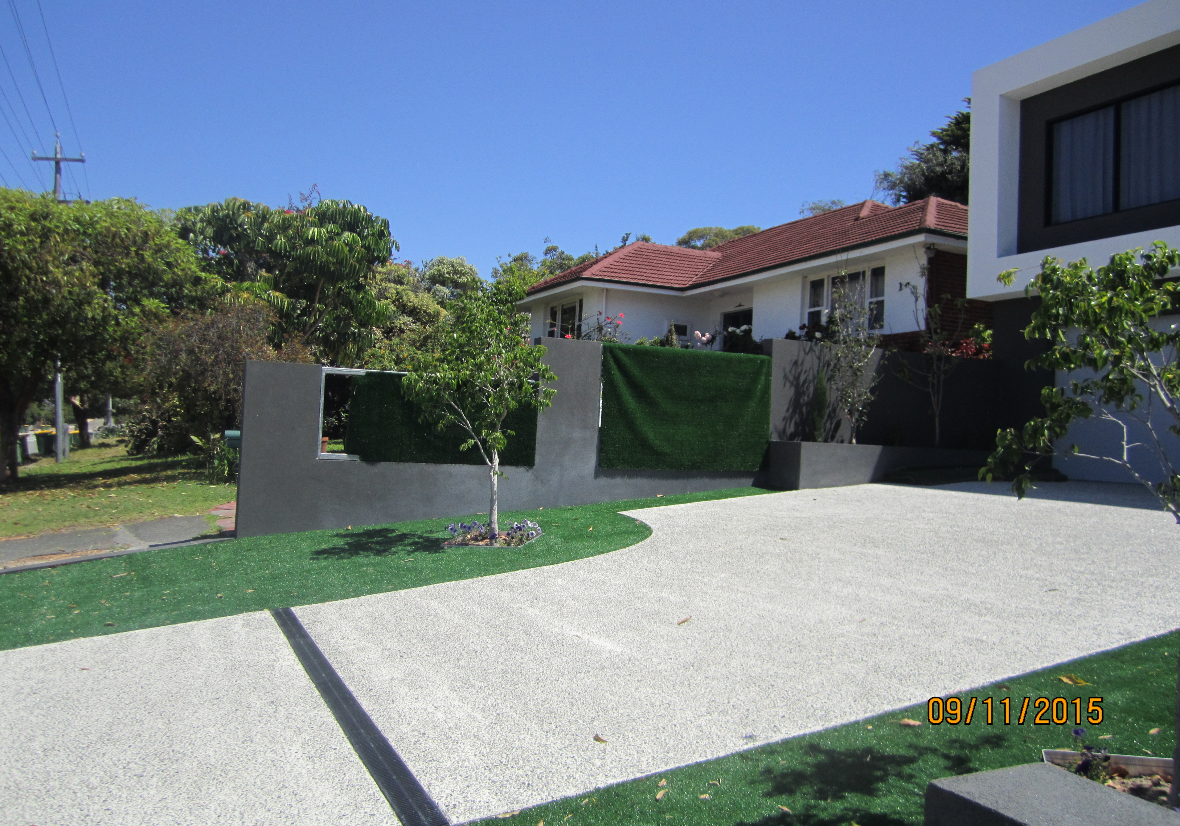
PD54.15 Attachment 6 - Existing fencing and solid infill panels facing 149 Rochdale Road
