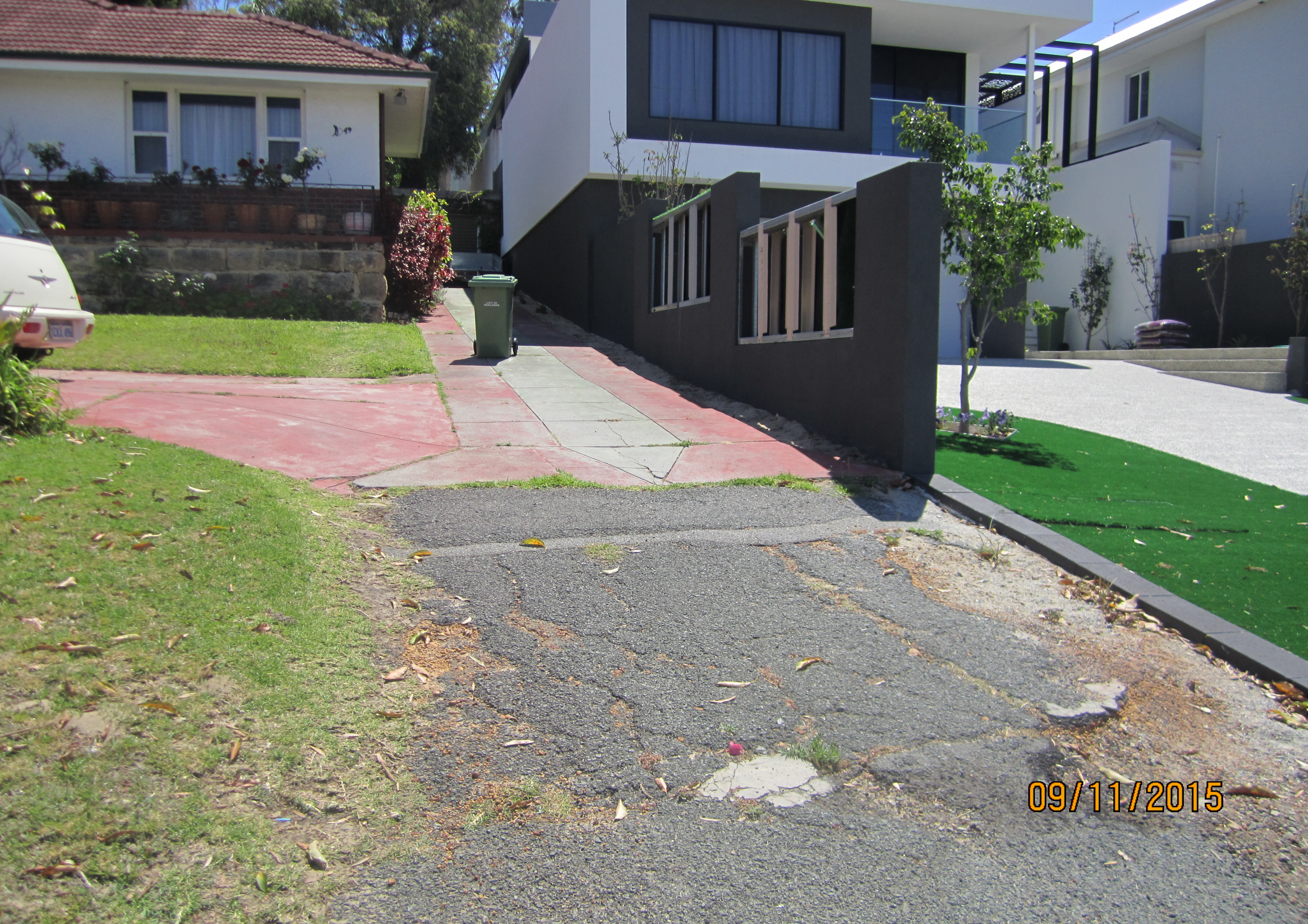
PD54.15 Attachment 8 - Existing driveway at 149 Rochdale Road
