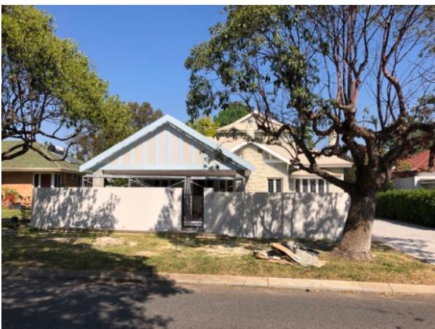
75 Dalkeith Rd Currently under construction ~2m from front boundary
