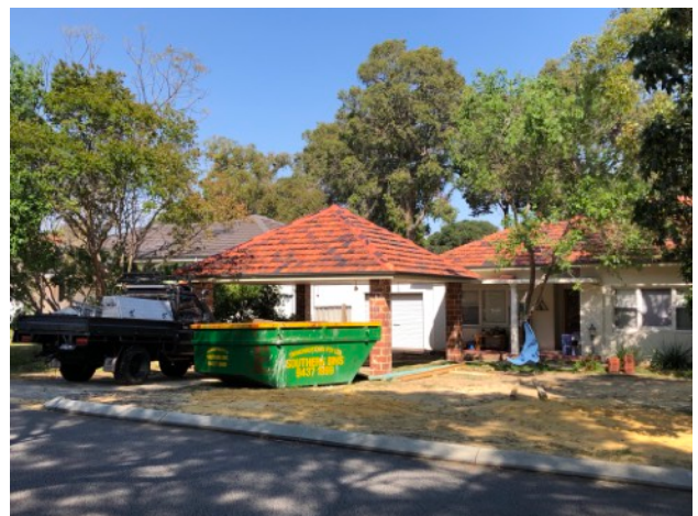
117 Dalkeith Rd Currently under construction ~1-2m from front boundary
