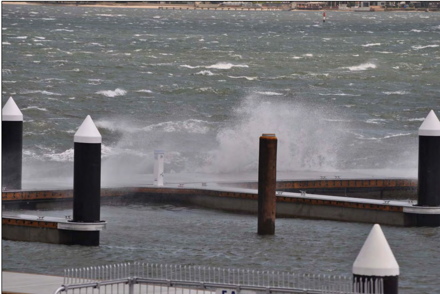
Figure 6 : Bellingham Attenuator preventing Wave Damage
