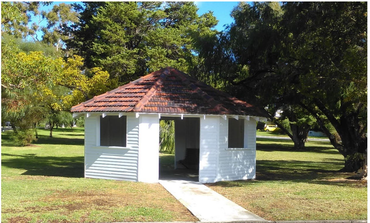
Figure 3: External refurbishment - April 2018
