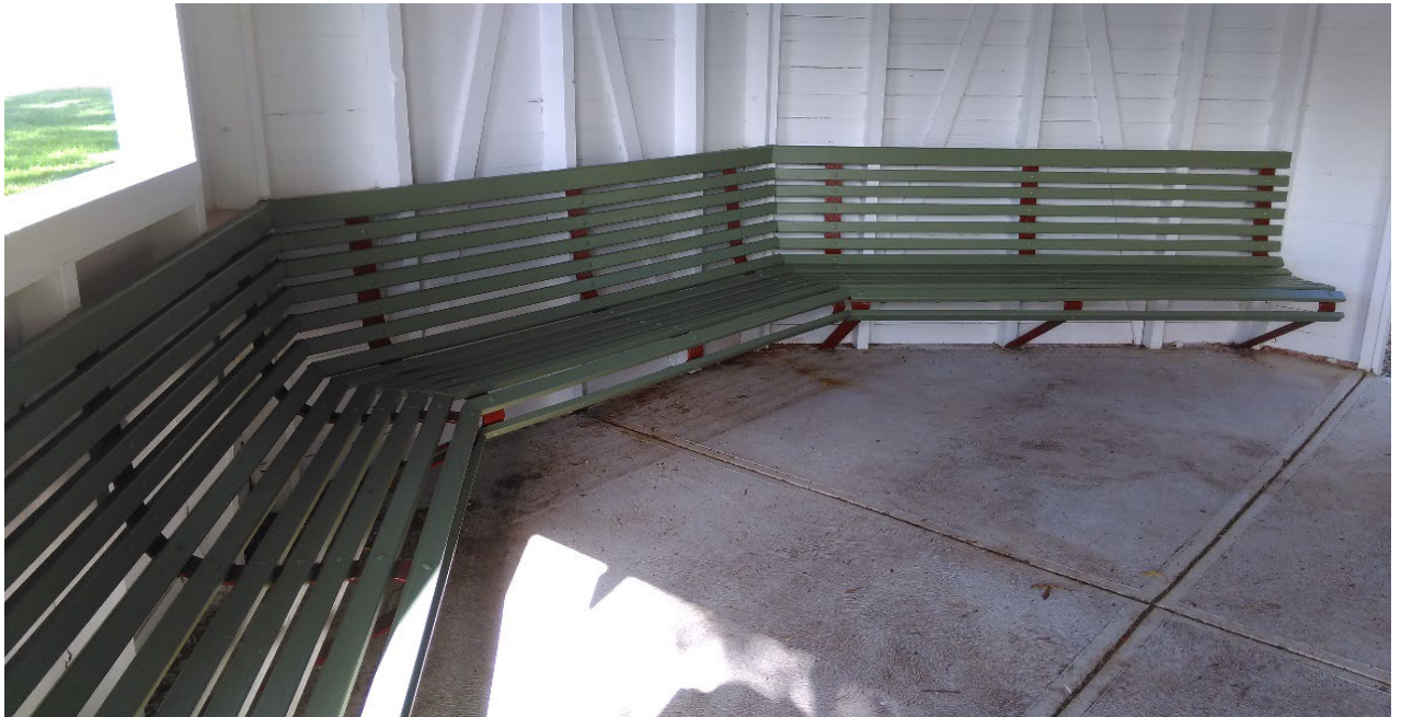
Figure 2: Internal refurbishment - April 2018
