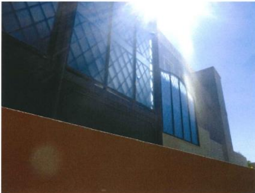
Photograph 1: Two-storey elevated outdoor living area constructed on No. 132 Victoria Avenue and adjoining the retained area along the northern boundary of the subject site. View from the paved area adjoining the laundry, looking north-east.
