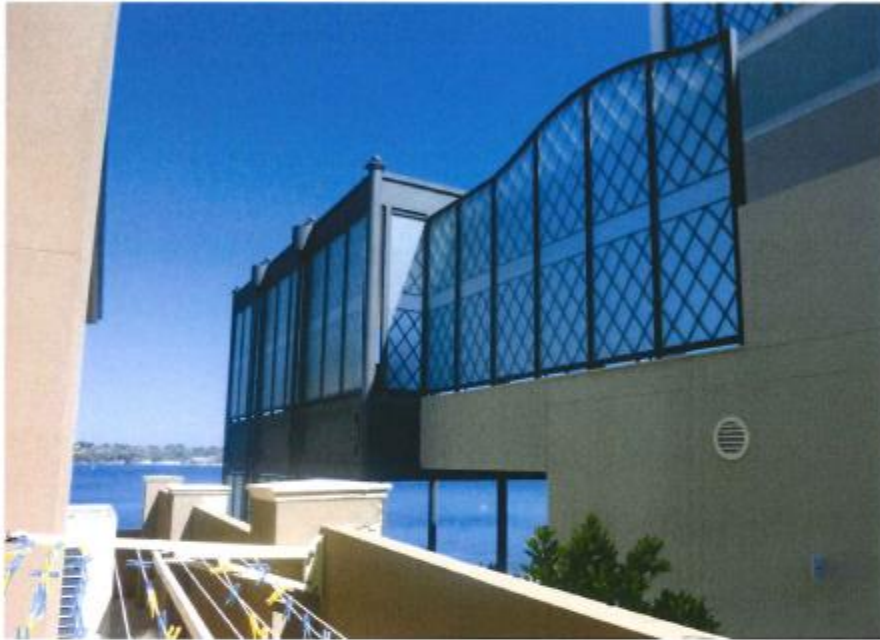
Photograph 2: Two-storey outdoor living area on adjoining No. 132 Victoria Avenue. Photograph shows the relationship between the retained area along the northern boundary of the subject site and the adjoining property, looking west.
