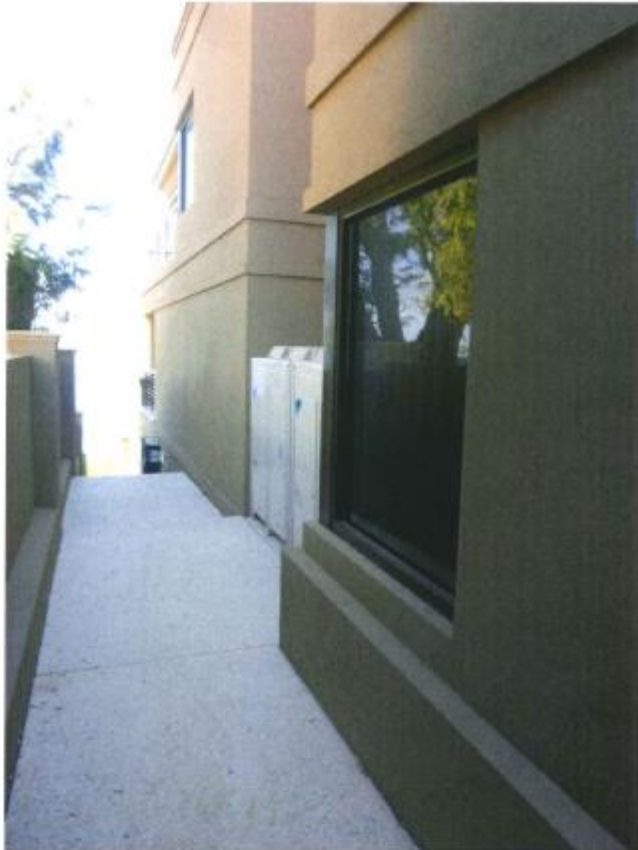
Photograph 12: The air conditioning units along the southern boundary are setback more than 2.0m from the boundary and are located behind and below the dividing fence.
