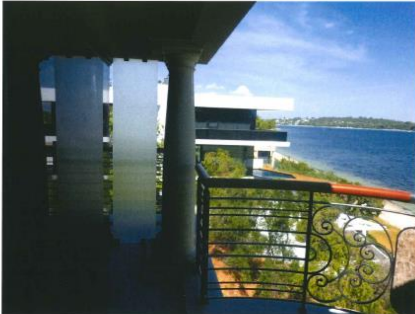
Photograph 11: The southern elevation of the upper floor balcony has been fitted with a 1.65m high obscure screen to restrict the cone of vision into No. 138 Victoria Avenue.
