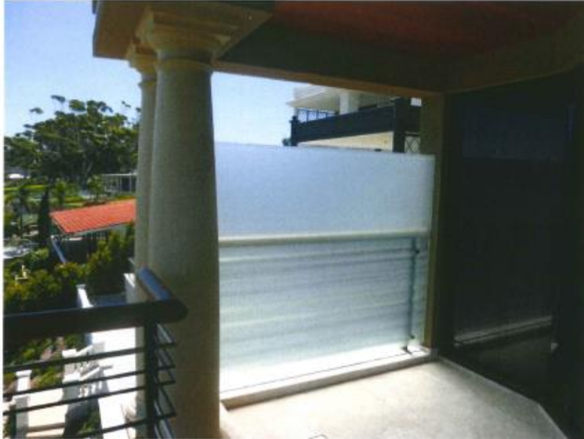
Photograph 9: The northern elevation of the Upper Floor balcony has been fitted with a 1.65m high obscure screen to restrict views within the cone of vision at No. 132 Victoria Avenue.
