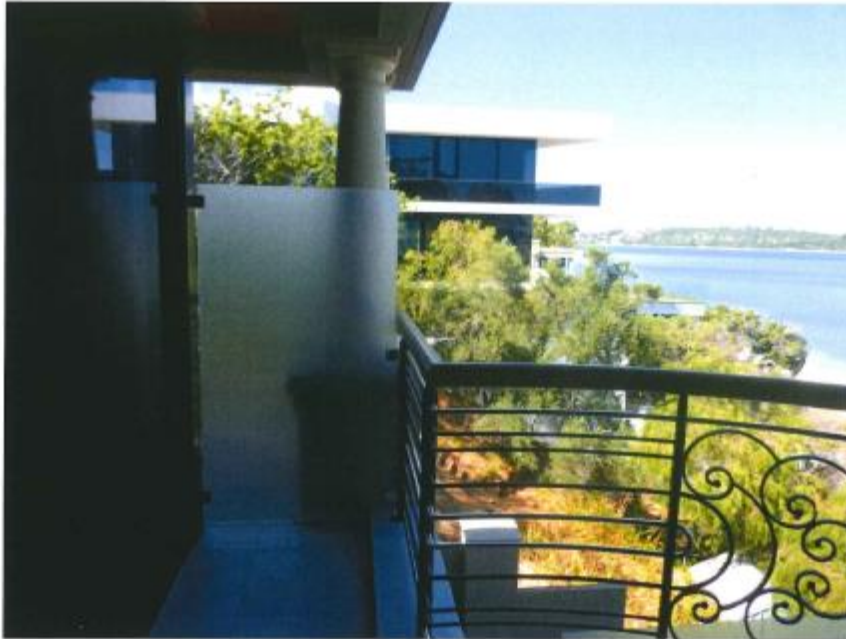
Photograph 10: The southern elevation of the ground floor balcony has been fitted with a 1.65m high obscure screen to restrict the cone of vision into No. 138 Victoria Avenue.
