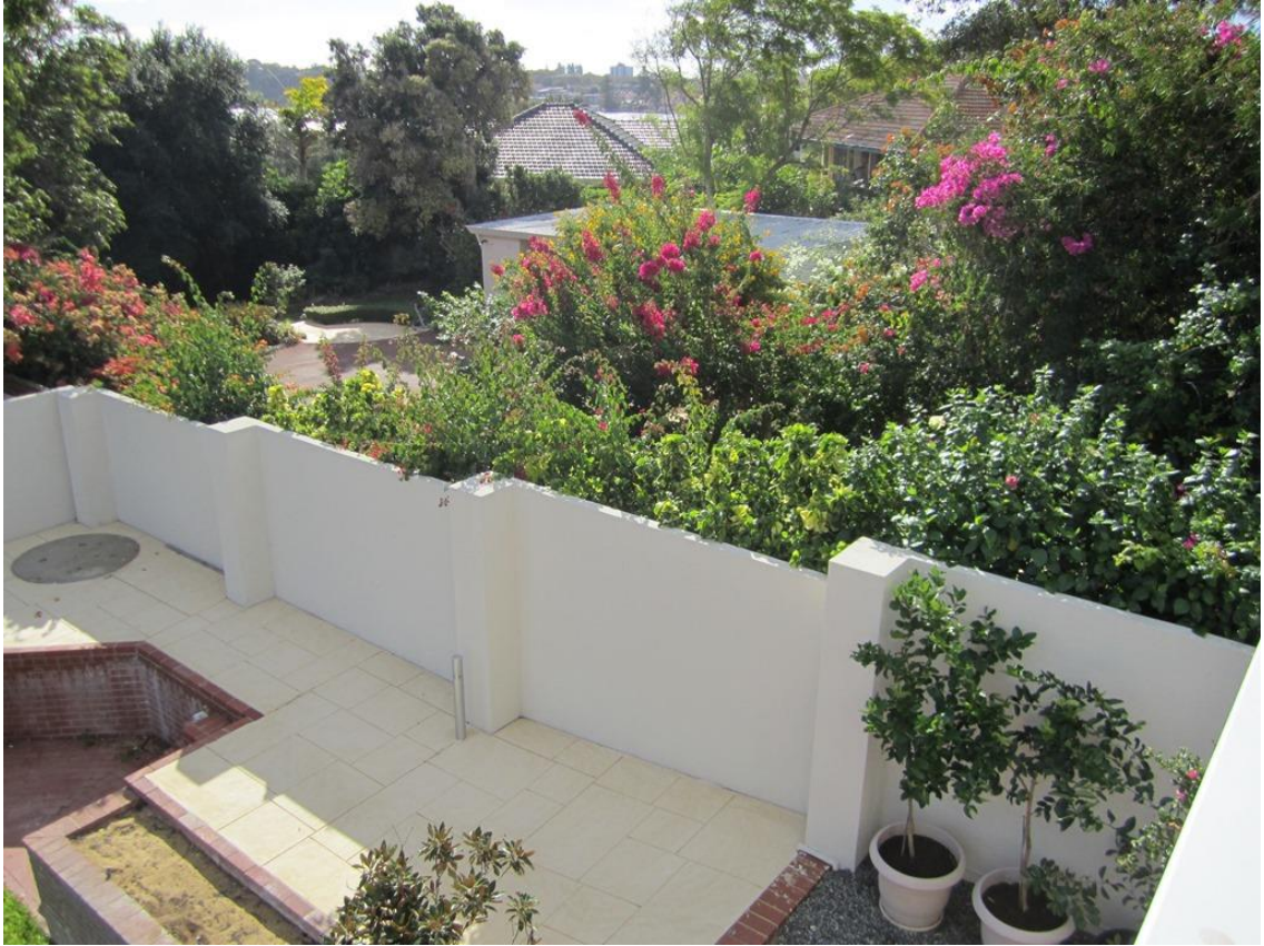
Site (Rear Yard, Northwest) – Retaining Walls, Landfill and Over-Height Fences
