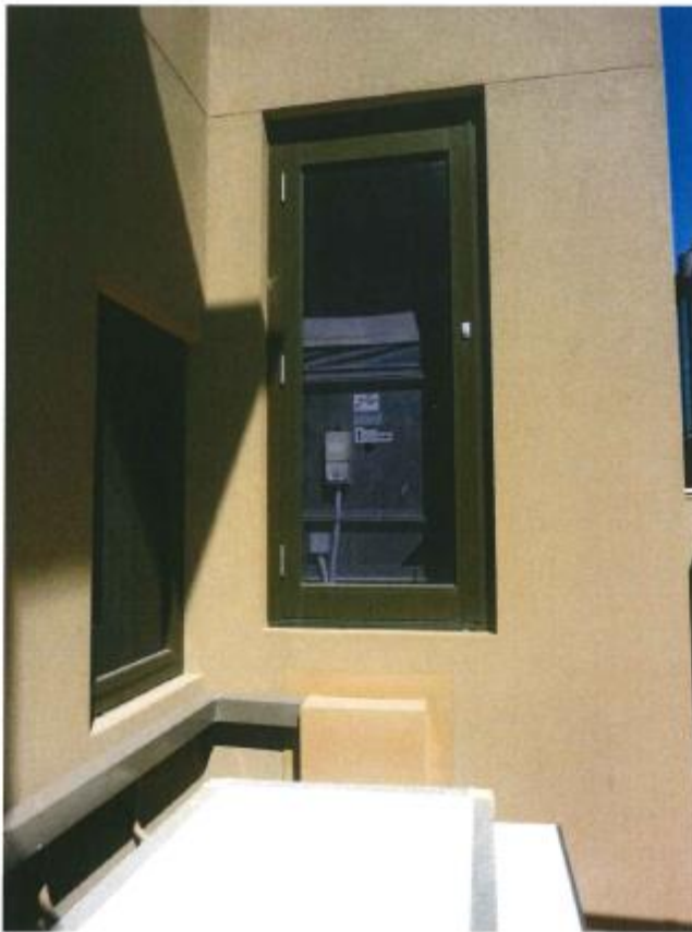
Photograph 8: An additional "wall" was created by enclosing the air conditioning infrastructure located along the northern side of the dwelling. Enclosing the infrastructure has screened it from view and removed any potential for noise disturbance to the adjoining property.
