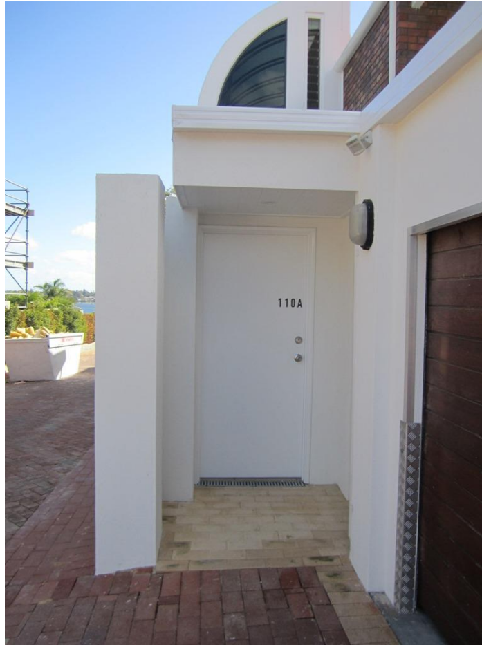
Site (South) – Modified Portico
