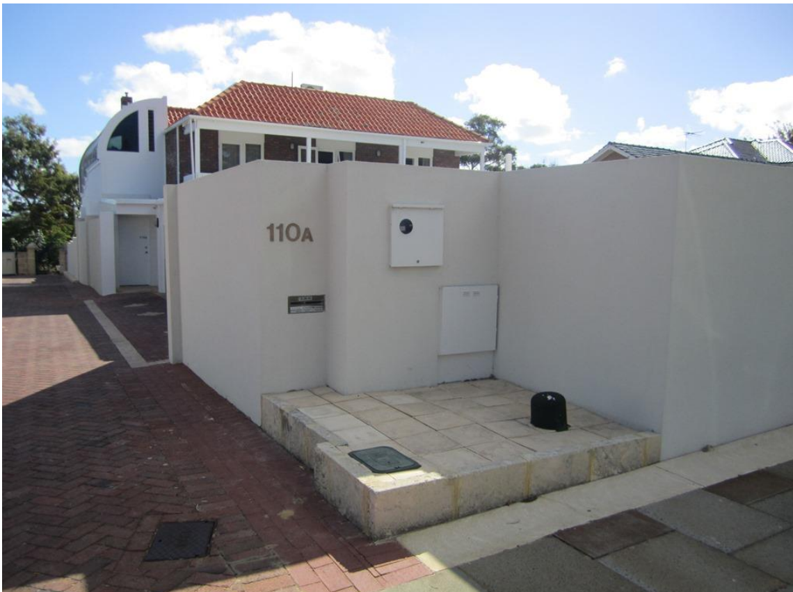
Site (Southeast) – Modified Corner and Additional Height of the Front Fence
