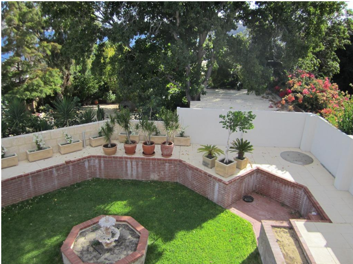
Site (Rear Yard, West) – Retaining Walls, Landfill and Over-Height Fences
