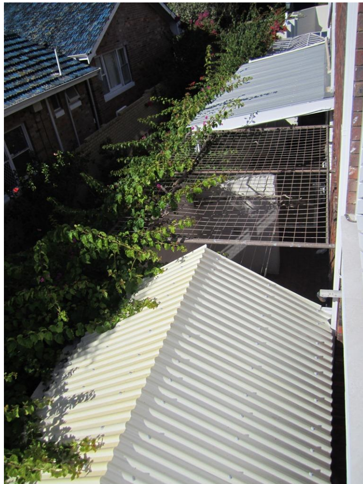
Site (Side Yard, Northeast) – Patios and Pergola
