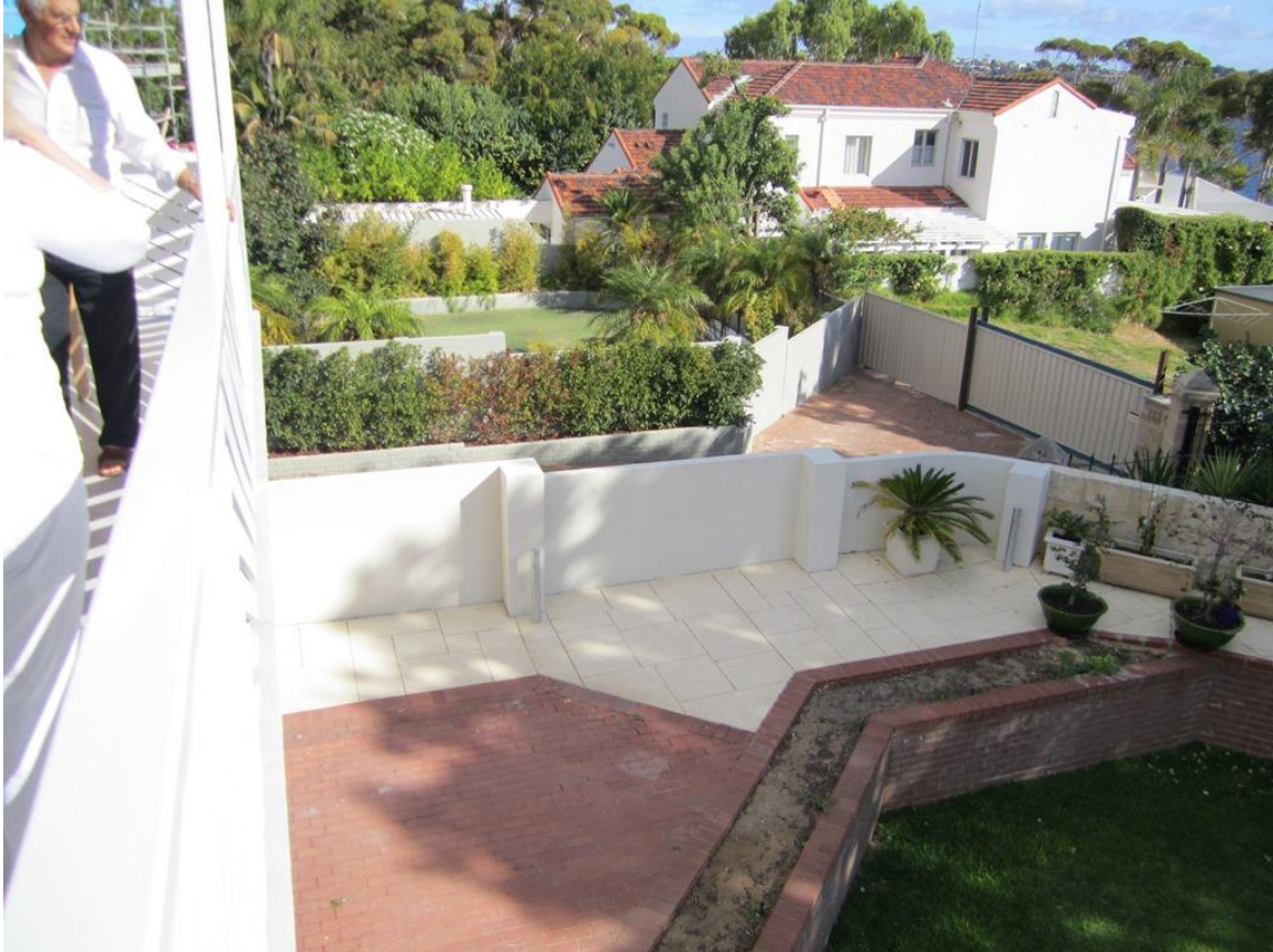
Site (Rear Yard, Southwest) – Retaining Walls, Landfill and Over-Height Fences
