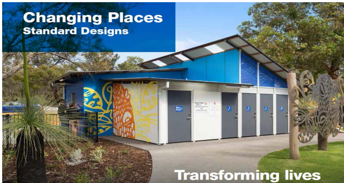
Figure 1: Landmark Changing Places Facility
