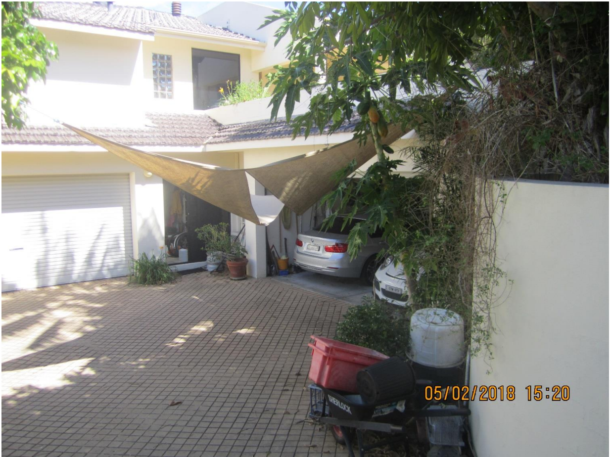
Photo 7 – Existing garages proposed to be converted
