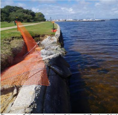
Figure 1 - Collapsed section of river wall (October 2016)
