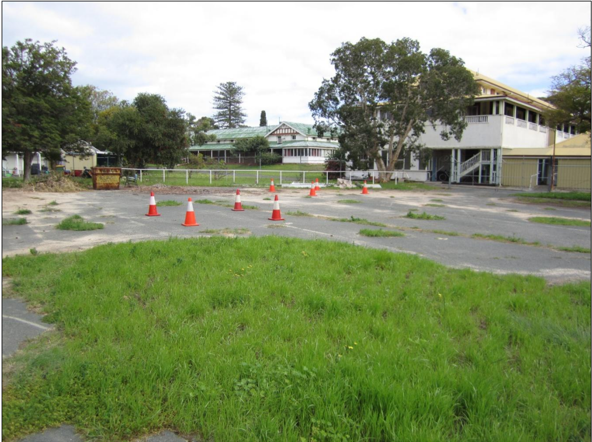
Physical Obstruction to Car-Parking Bays – Unserviceable Condition
