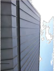
Metal Cladding to architect's selection Colorbond Matt Finish
