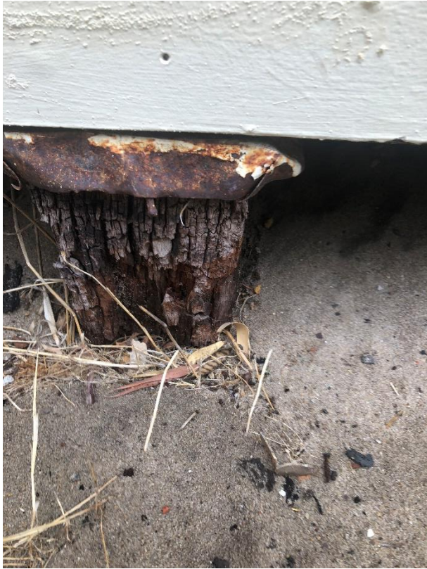
Photograph 12 – Damaged Timber Stump
