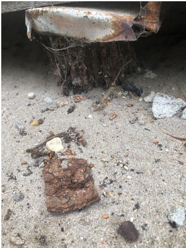
Photograph 11 – Damaged Timber Stump
