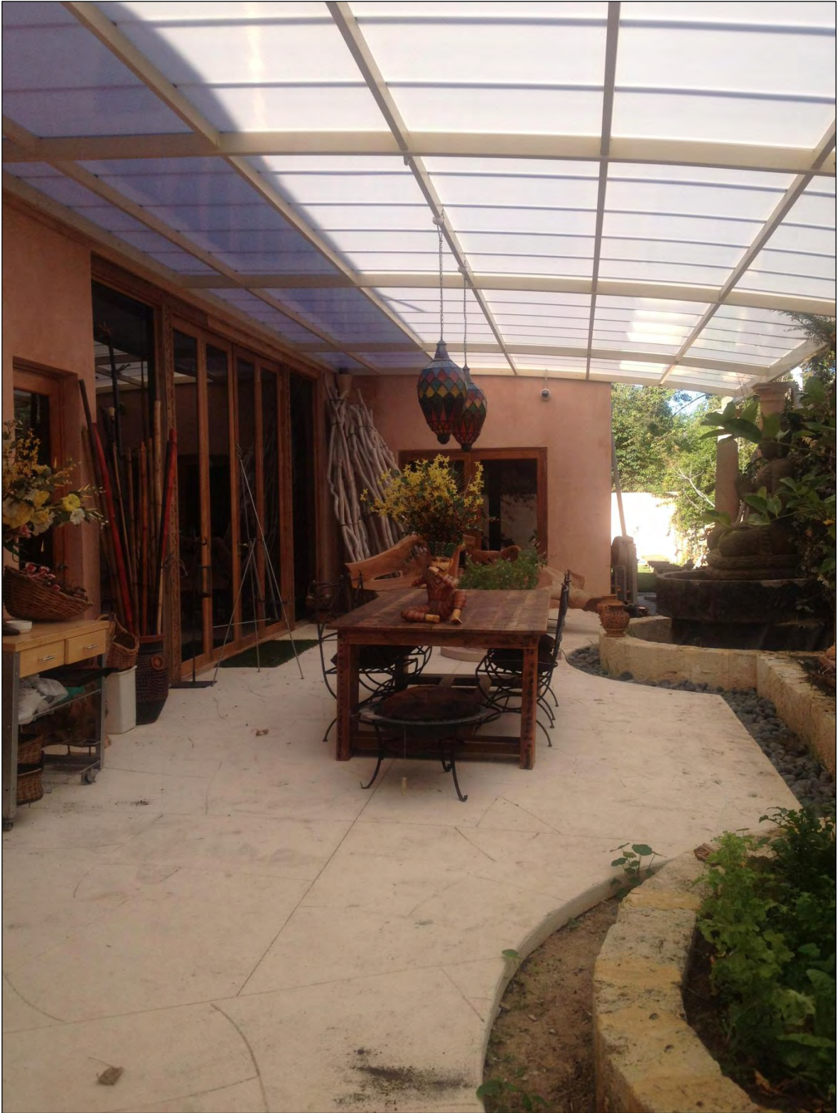
Unretained Raised Levels (West)
