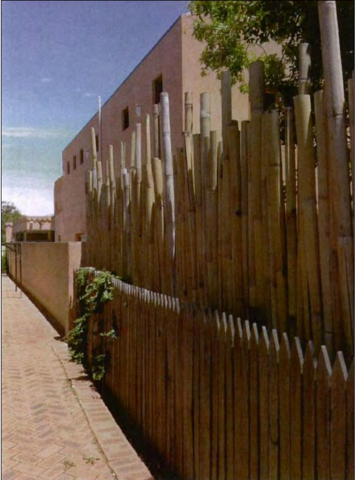
Over-Height Dividing Fence (East) from Neighbour's Side
