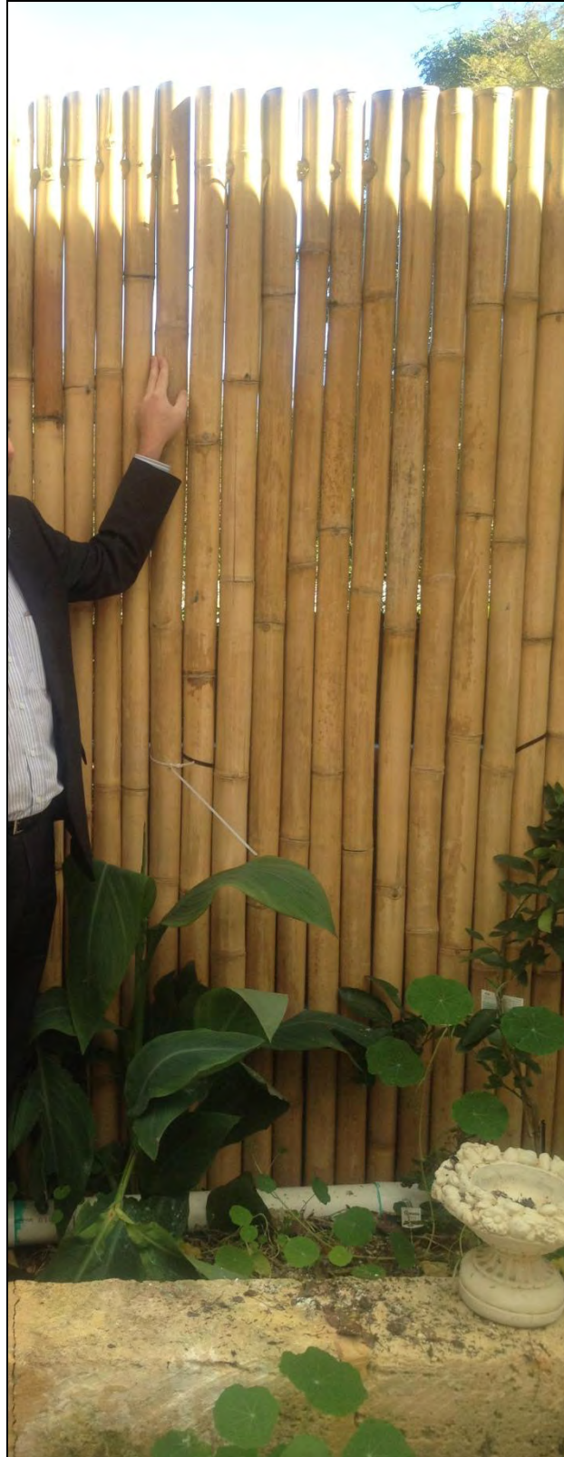
Over-Height Dividing Fence (West)
