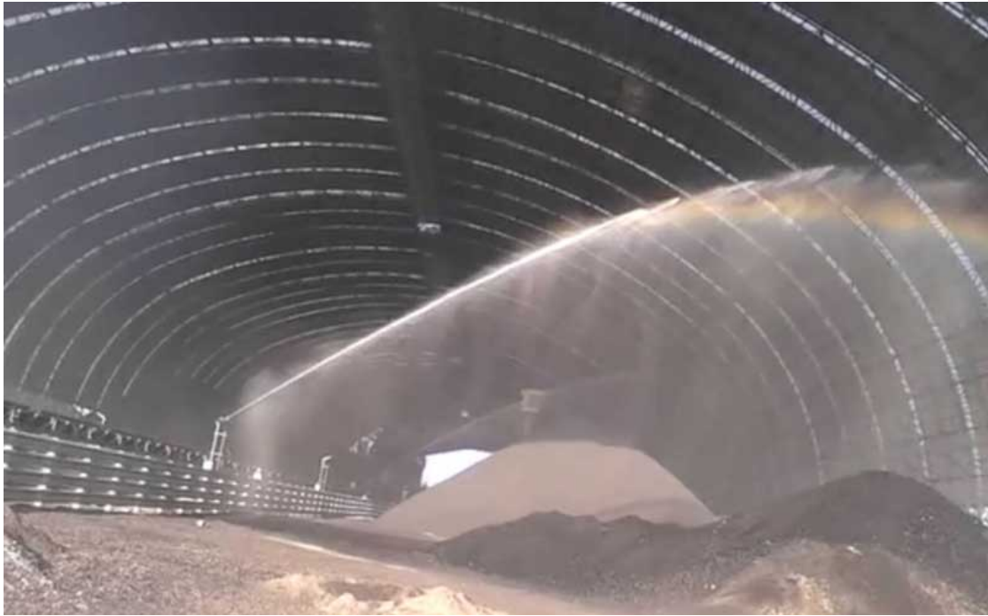
Example of dust control in municipal heaps
