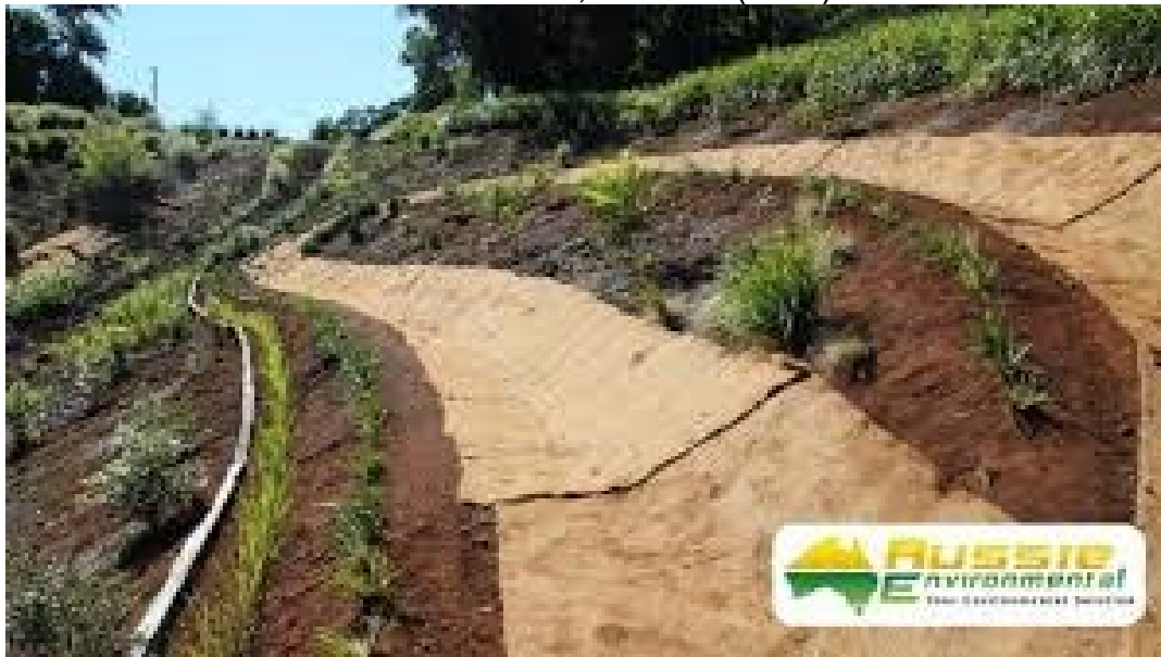
Example of combined dust control and slope re-generation
