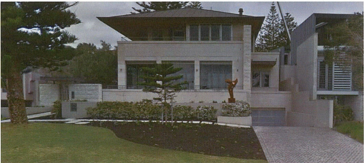
Figure 9: Street view of No. 24 Odern Crescent, Swanbourne.
