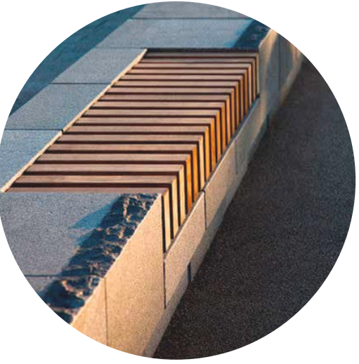
Composite Timber On Concrete wall
