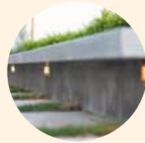
Concrete wall to entrance
