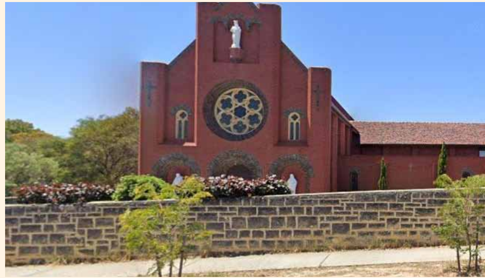
ORIGINAL LIMESTONE WALL AROUND CARMELITE CONVENT
