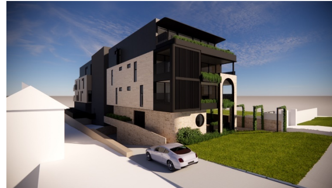
Concealed / Integrated Roof Design
