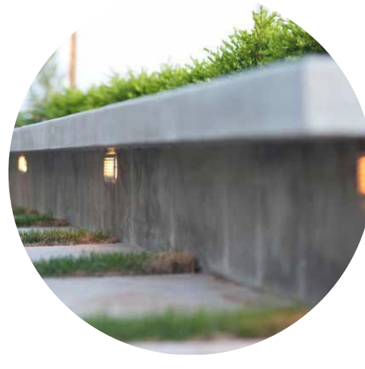
Concrete wall to entrance
