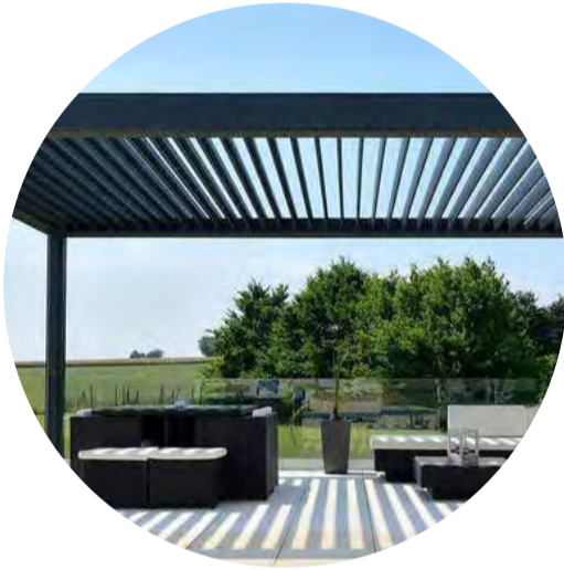
Shade structure on Rooftop
