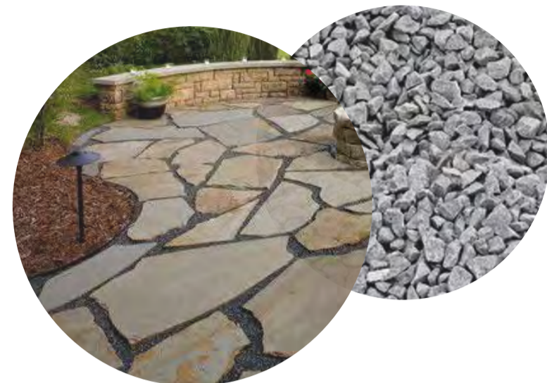
Gravel & flagstone paving to form cross lot link
