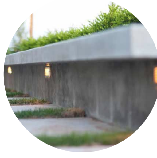
Concrete wall to entrance
