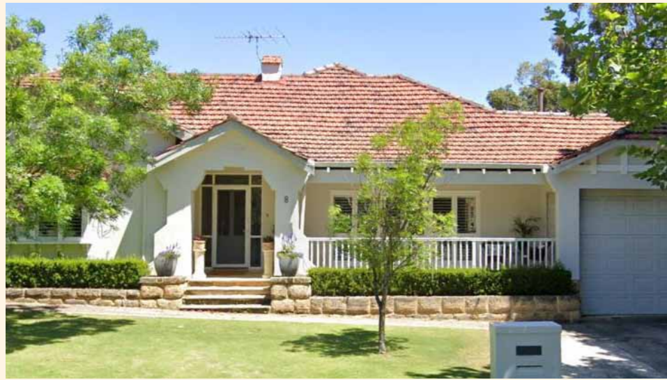
LIMESTONE FOUNDATION AT 8 EDNA ROAD
