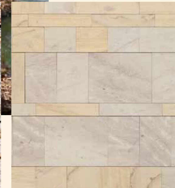
LIMESTONE TILE CLADDING
