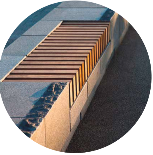
Composite Timber On Concrete wall
