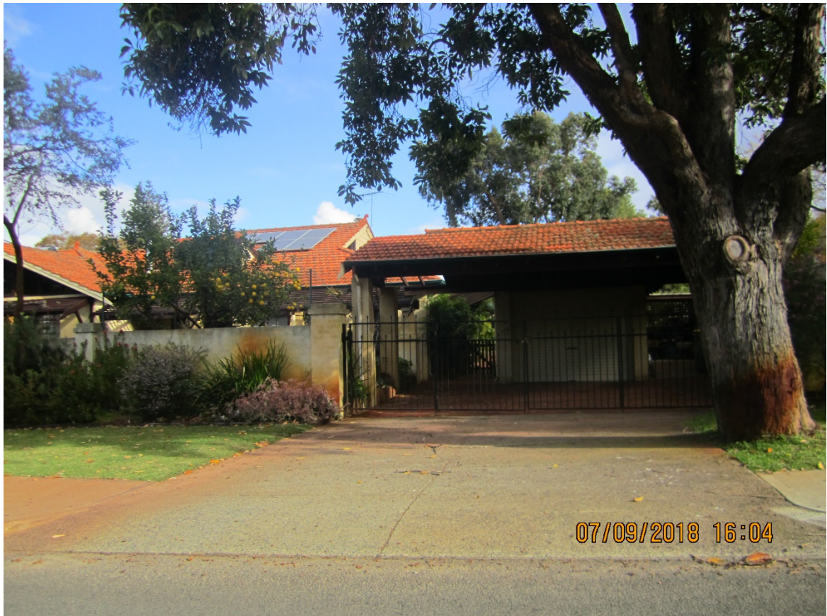
33 Portland Street, Nedlands – carport setback over 1.5m to Gordon Street
