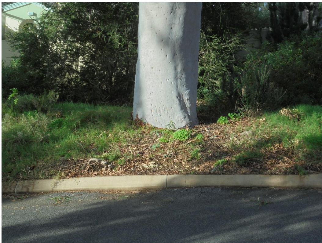
Figure 3 Displaying the base and lower trunk of Tree 1 viewed from the northern side.
