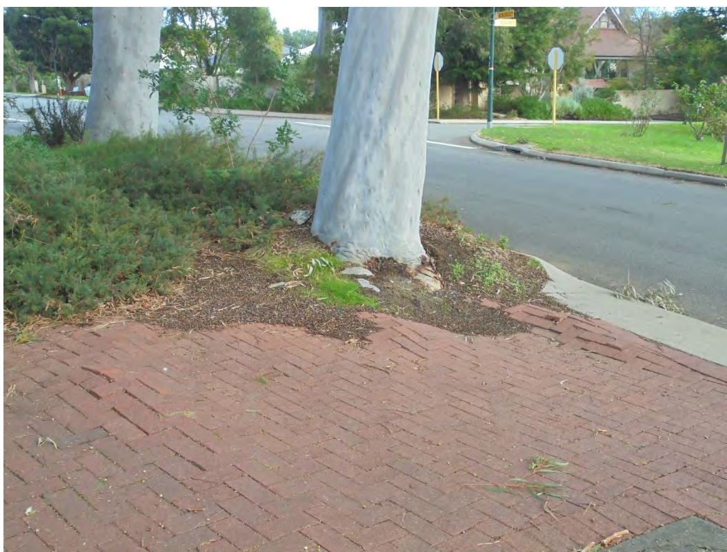
Figure 4 Displaying the base and lower trunk of Tree 2 viewed from the eastern side with lifting of adjacent paving evident.
