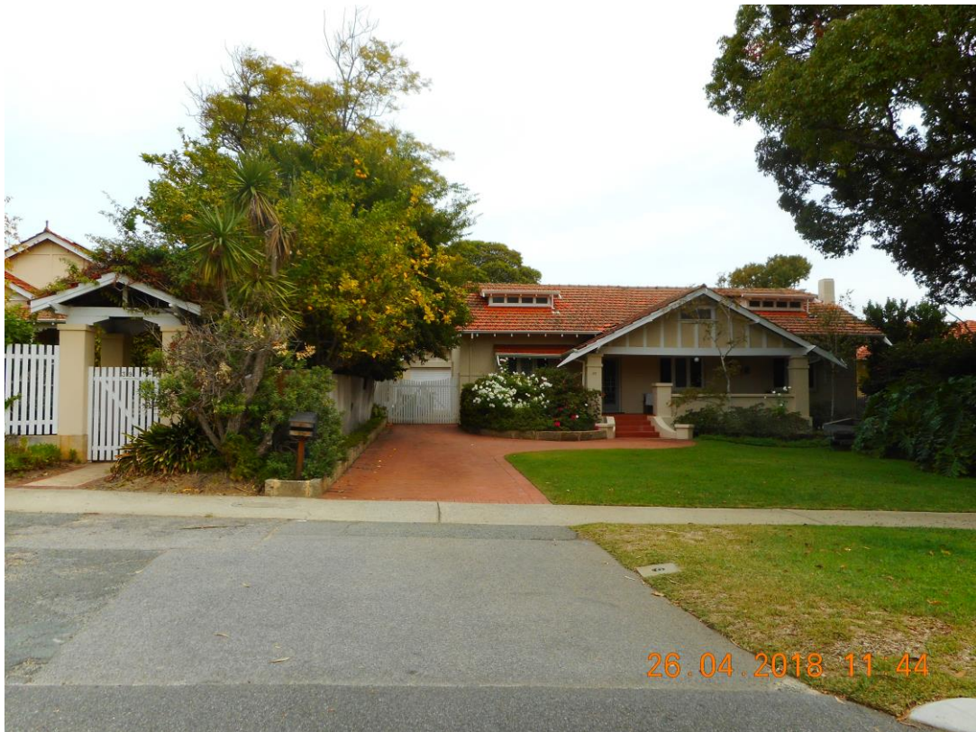
Below – View of the subject property as seen from Tyrell Street
