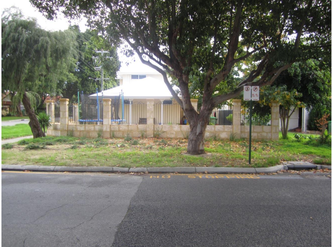
Site – Front (East)
