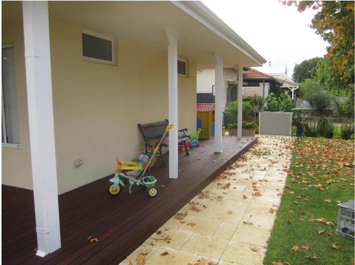
Site – Decking & Air-Con
