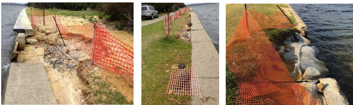
Figure 2: Typical River Wall Degradation
