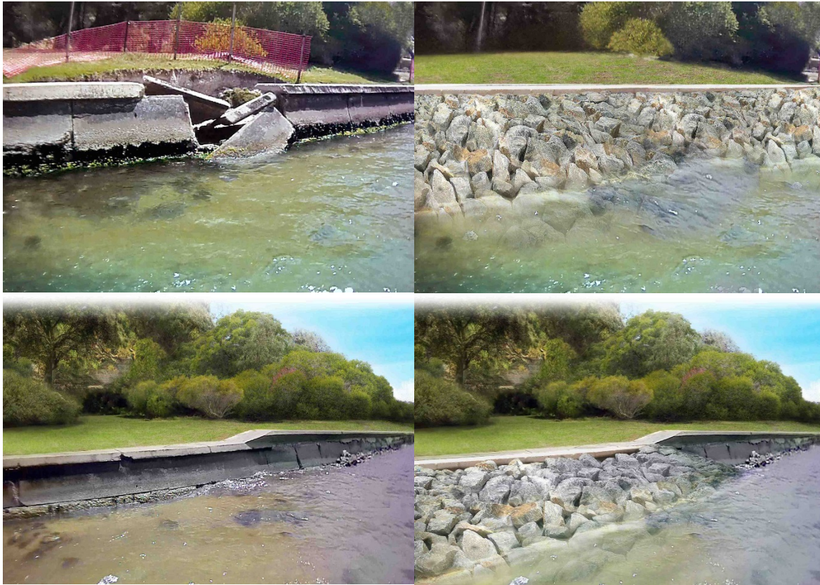
Figure 5: River Wall Before (left) and After (right)
