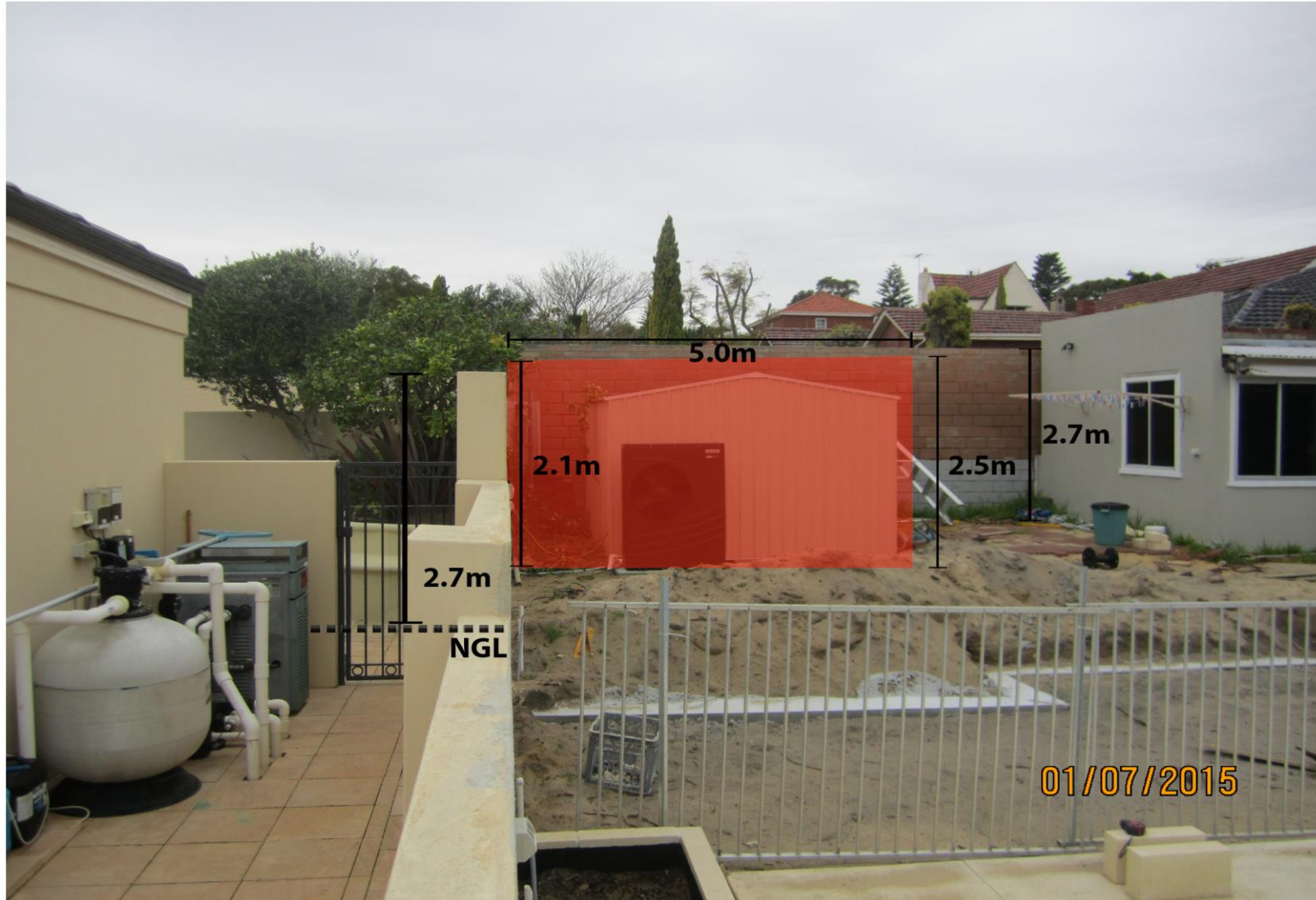
View from dividing fence line showing the differing natural ground levels (dashed)
