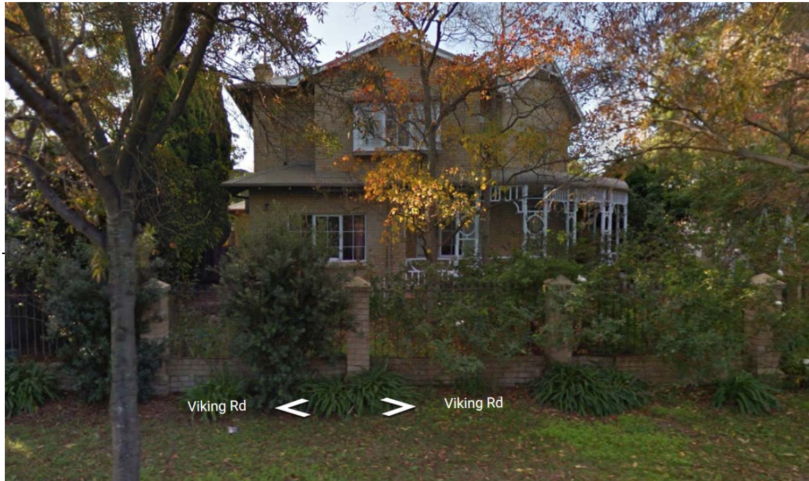
Photograph 1: Street elevation of No. 15 Viking Street, Dalkeith. Pine trees located to the left of the existing dwelling screen the proposed wall.
