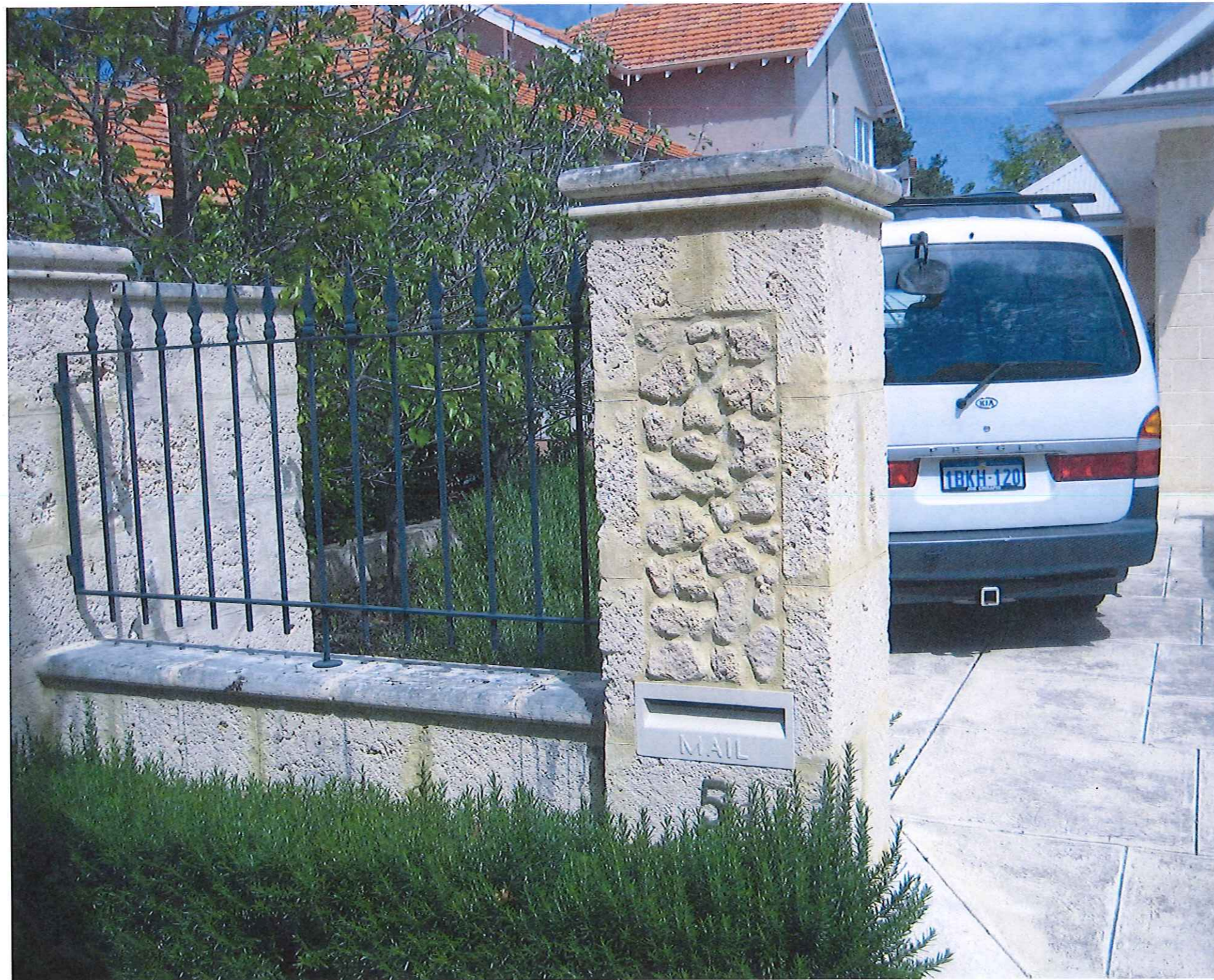
* FURTHER VIEW OF # 5 BURWOOD STREET 7/10/14
