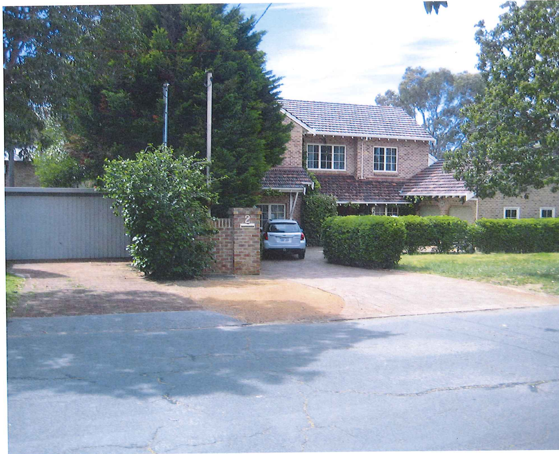
* FURTHER VIEW OF #2 BURWOOD STREET 7/10/14
