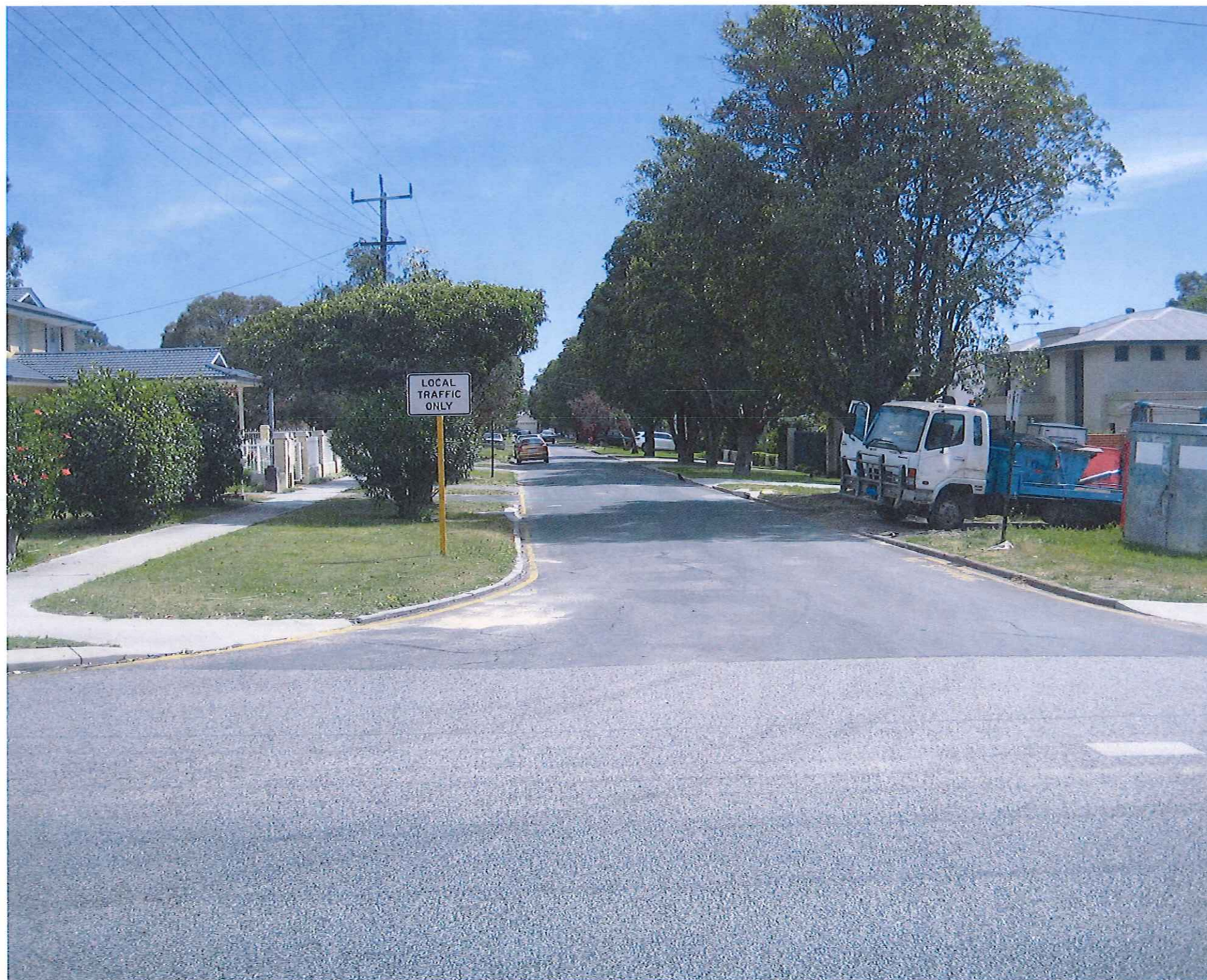
*VIEW NORTH ALONG BURWOOD STREET DEPICTING STREETScape (SUBJECT SITE IMMEDIATELY ON RIGHT). 7/10/14
