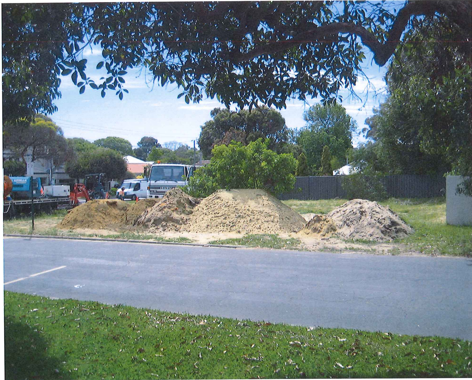
*FURTHER VIEW OF #57 ABERDARE ROAD 7/10/14
