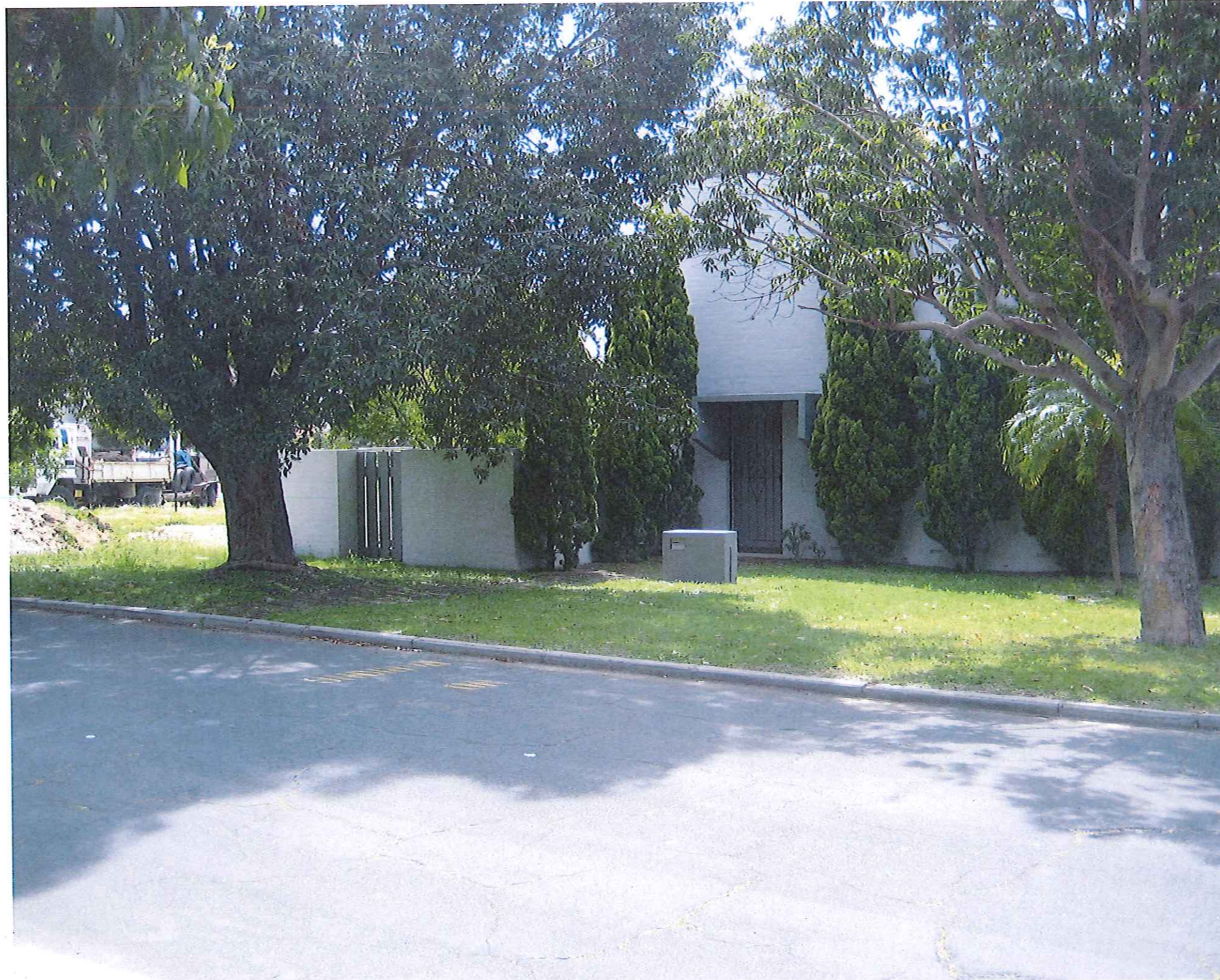
* VIEW OF # 57 ABERDARE ROAD (BURWOOD ST. FRONTAGE) 7/10/14
