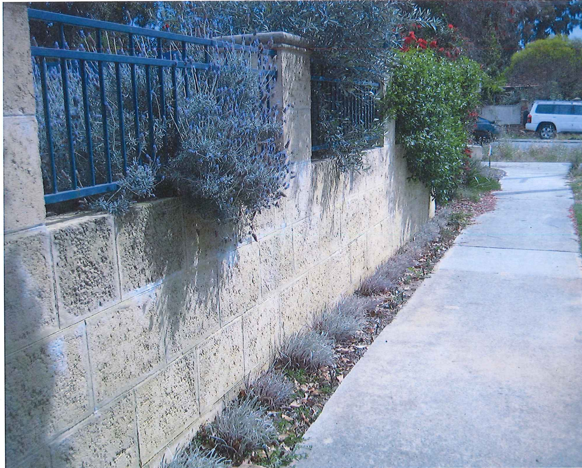
*FURTHER VIEW OF #59 ABERDARE ROAD 7/10/14
