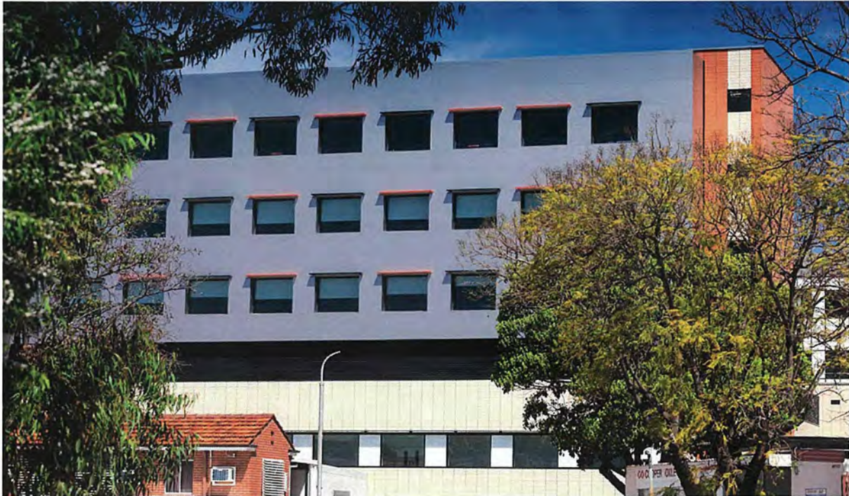
New Theatre & Ward Block (Anne Leach Wing) Completed 2015 Aluminium cladding and terracotta facade tiles
