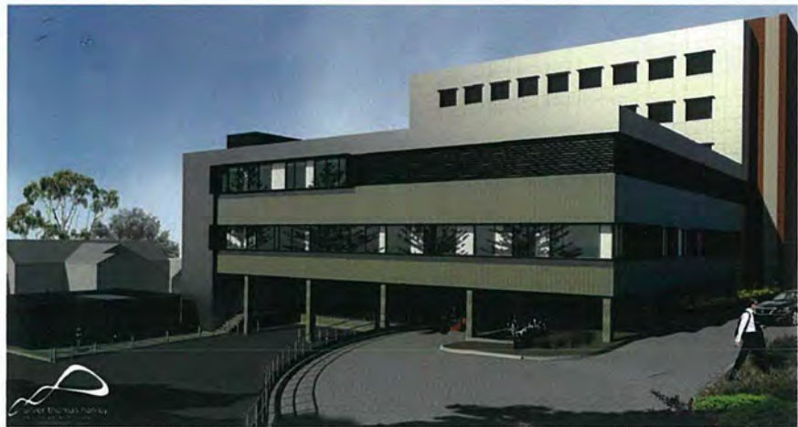
New Theatre Expansion (currently under construction)
