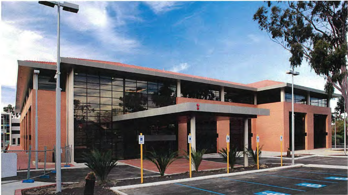
Medical Centre Completed 2009 Face brick, aluminium cladding, tinted glass
