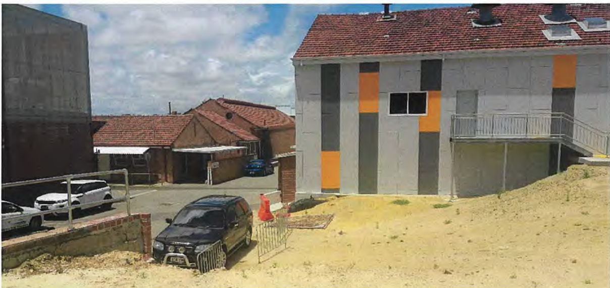
Old kitchen building stock Completed circa 1940s – being demolished
