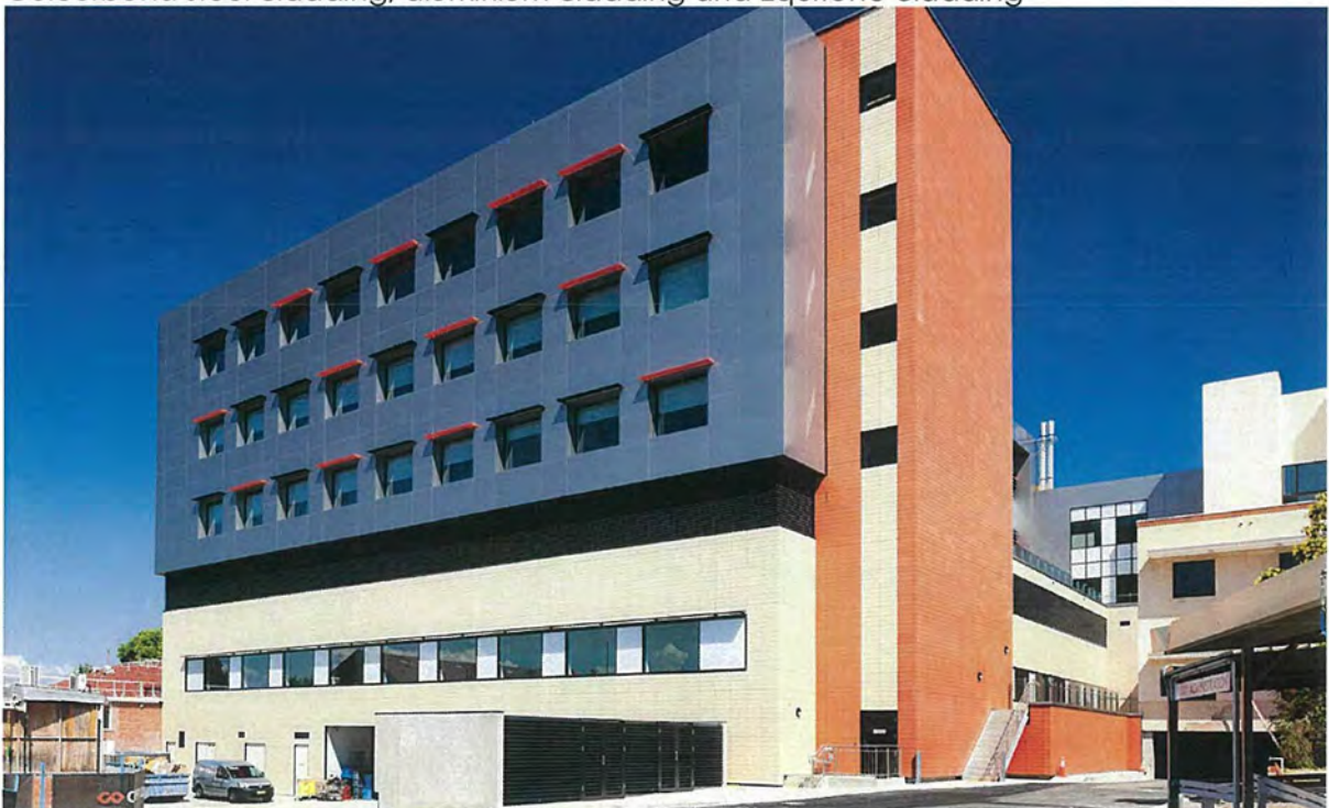
New Theatre & Ward Block (Anne Leach Wing) Completed 2015 Aluminium cladding and terracotta facade tiles
