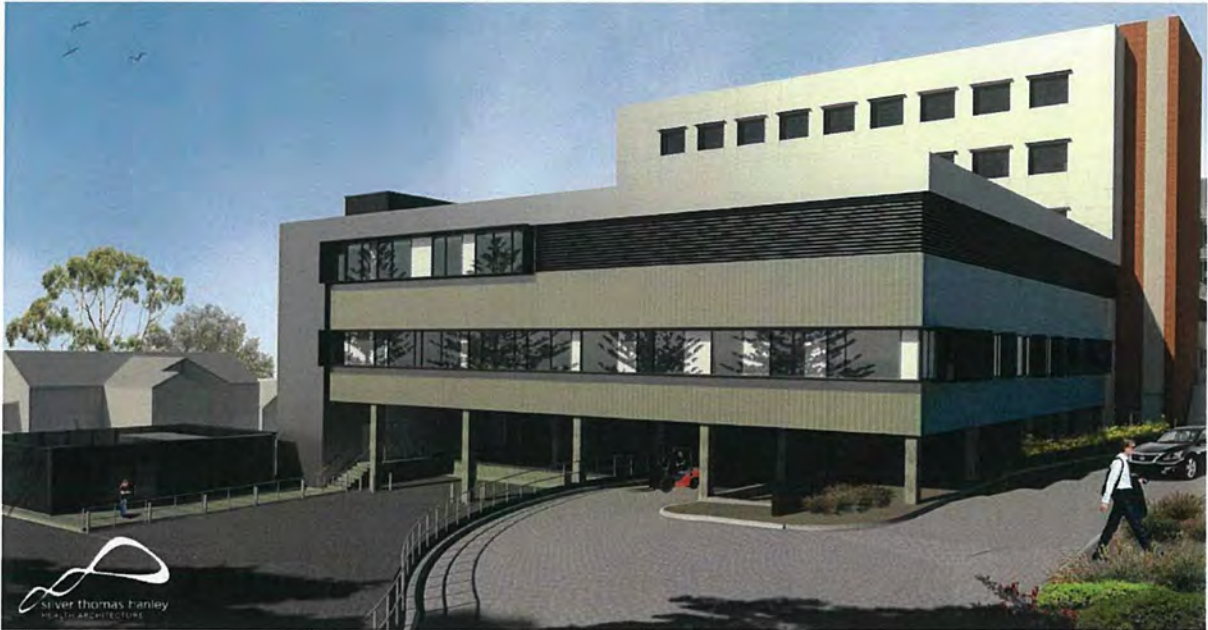
New Theatre Expansion (currently under construction) Colourbond steel cladding, aluminium cladding and Equitone cladding
