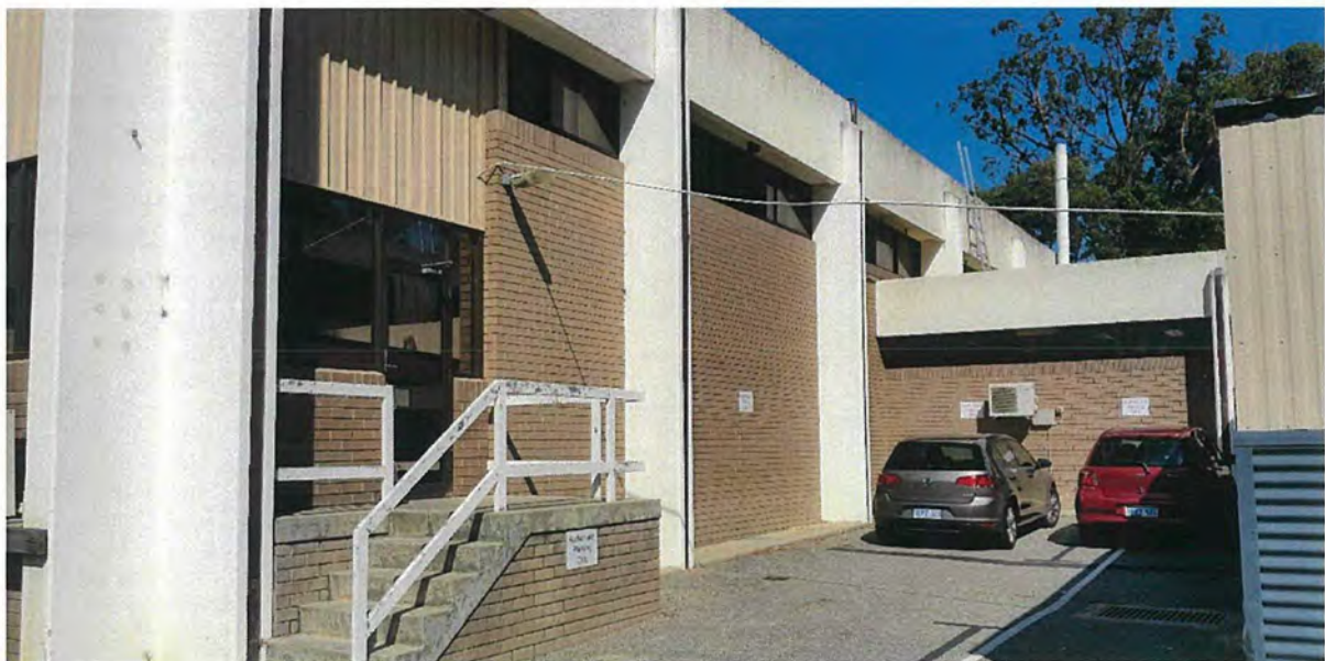
Old Administration building stock Circa 1980s – to be demolished long term Concrete, facebrick, render
