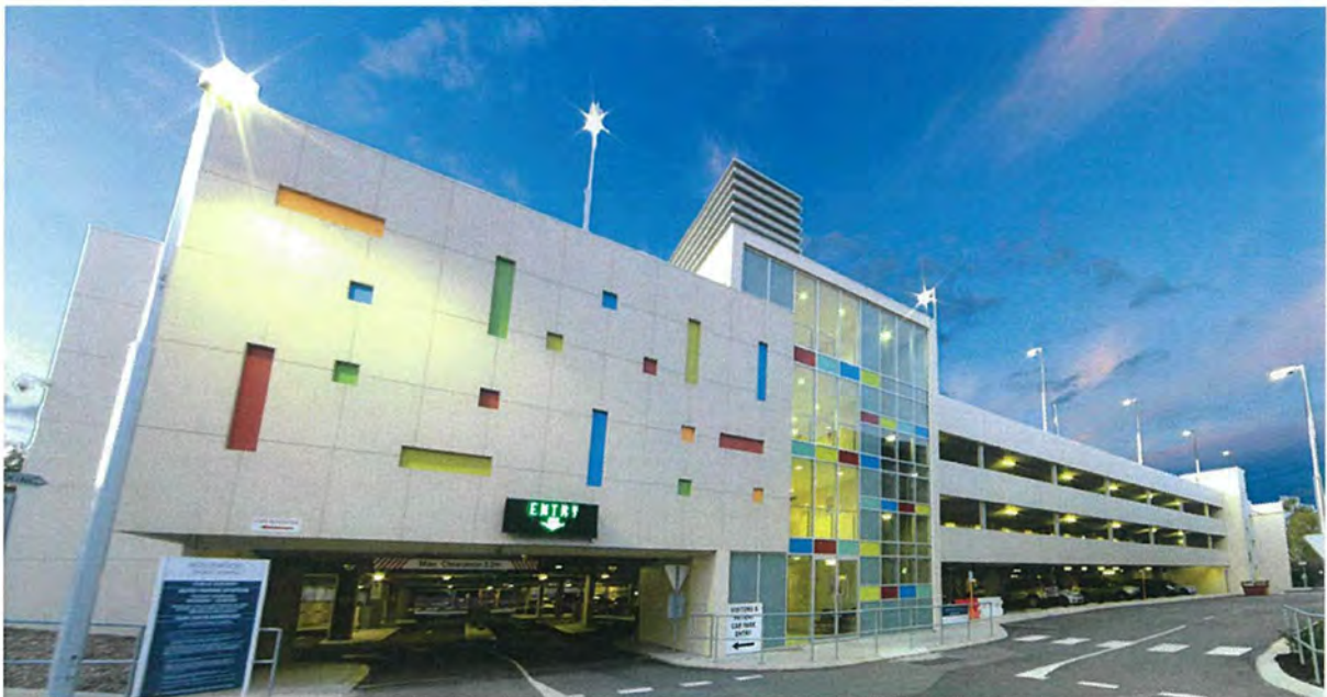
New Multi-Deck Parking Completed 2009 Painted concrete, CFC cladding and glass façade.
