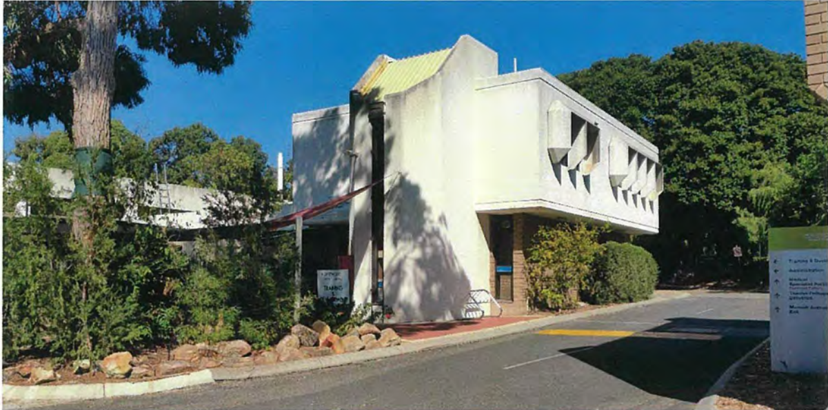
Old building stock Circa 1960s – to be demolished long term Concrete, facebrick, render
