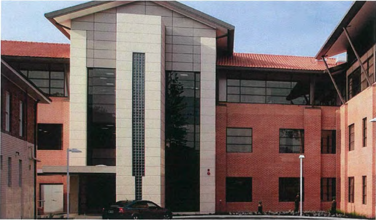
Marjorie Brislee Wing - Ward Block Completed 2009 Face brick, aluminium cladding, painted render, tinted glass
