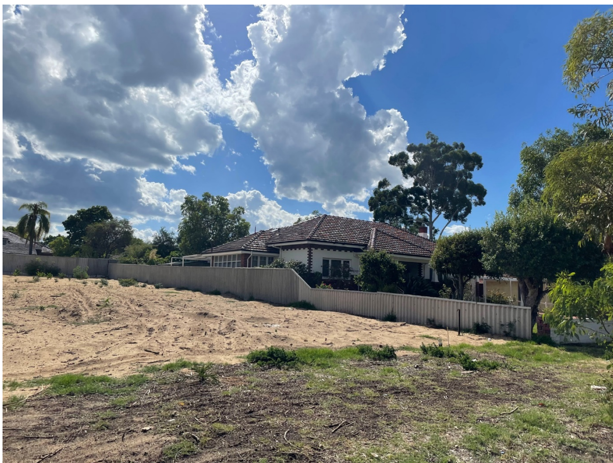
65 Dalkeith Road (LHS) and 63 Dalkeith Road (RHS)
