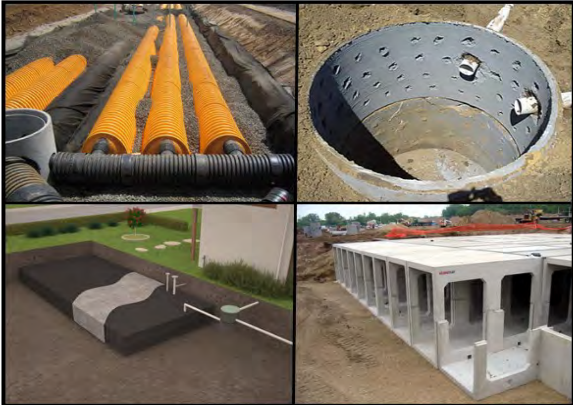
Figure 1: Common stormwater retention systems used in Western Australia (top left in a clockwise direction, StormTech SC-740, Soakwell, Atlantis Flo-Tank, StormTrap)
