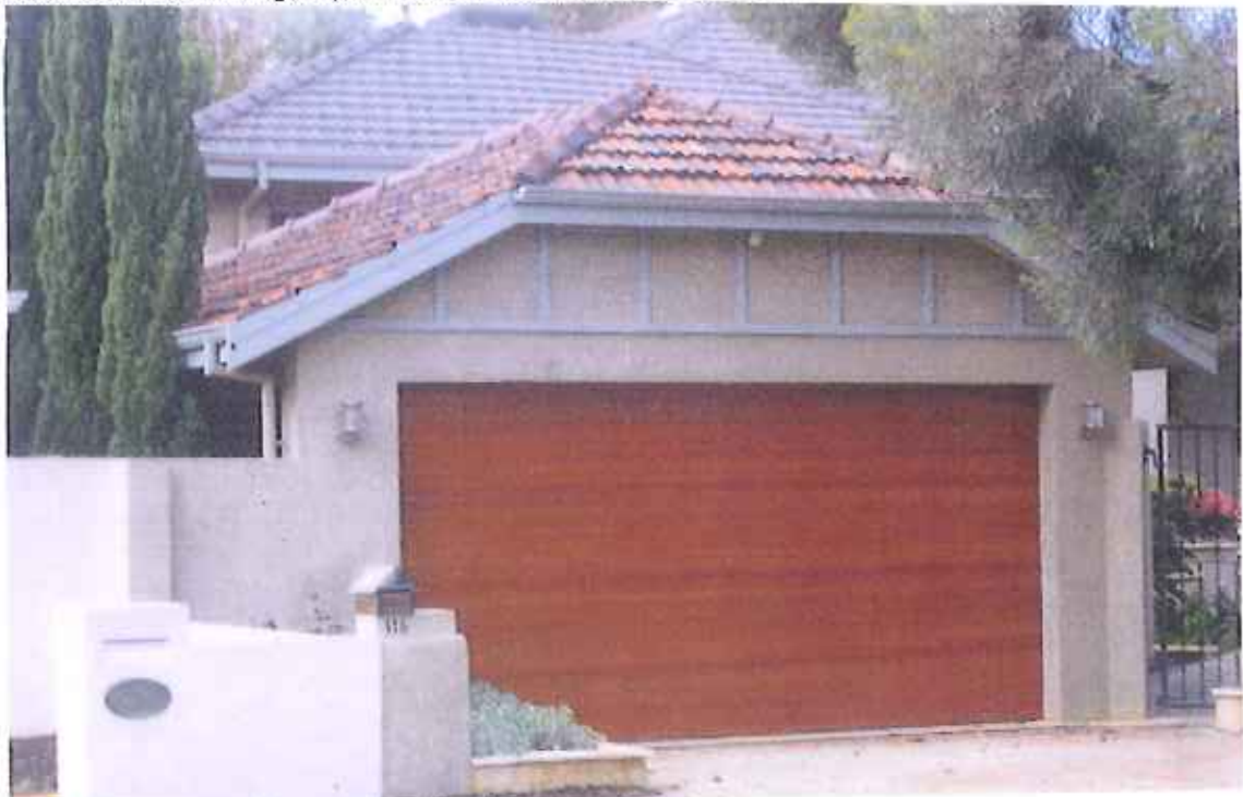
Picture above: Showing carport with solid garage door
