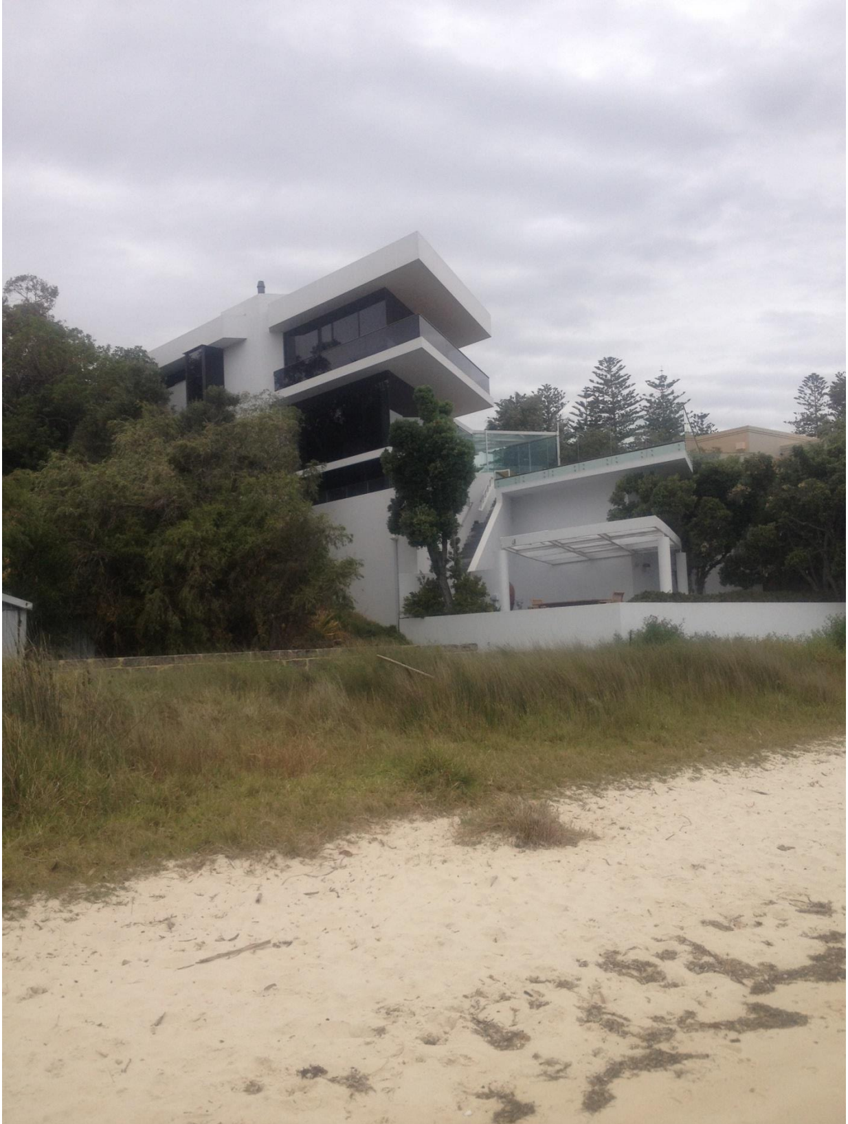
Neighbour (South) – Western Elevation
