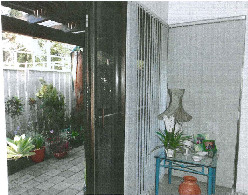
This shows how adjacent the framework is located to LIVING area of Unit 7/ 52 Weld St
