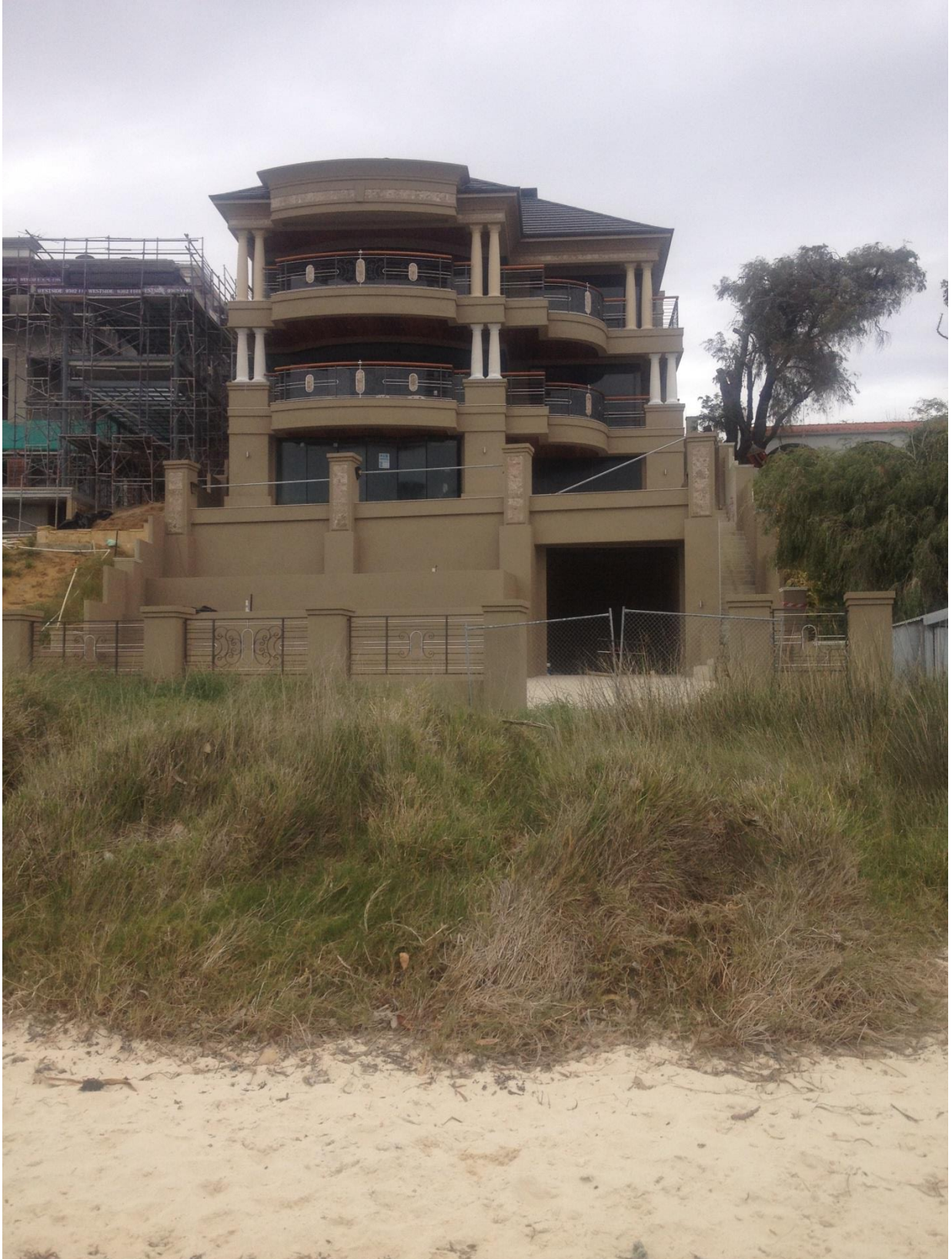
Neighbour (North) – Western Elevation
