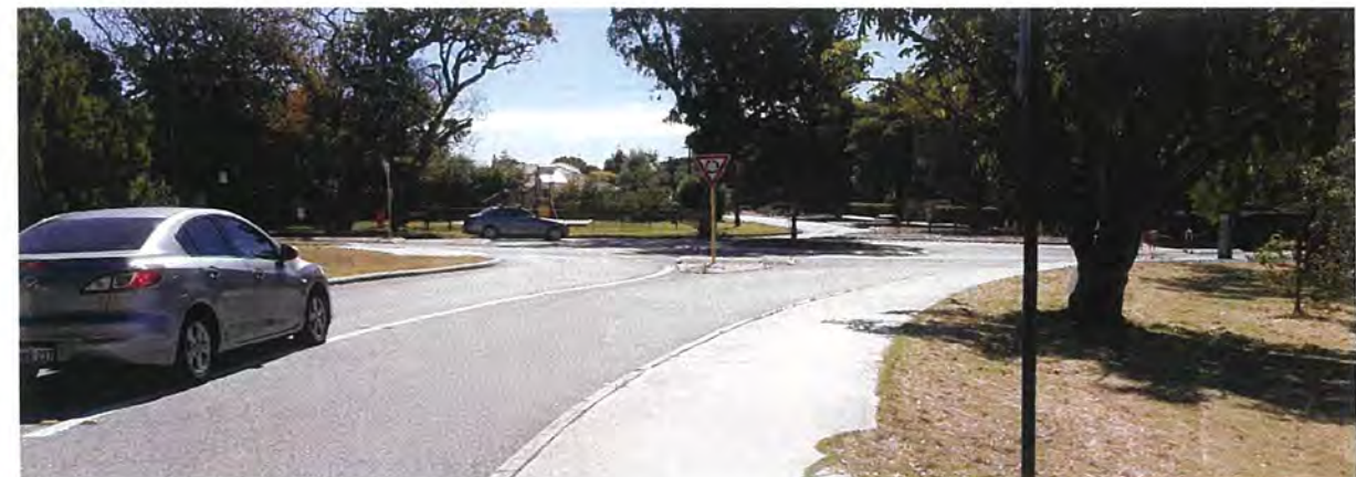
Figure 8: Roundabout intersection of Karella Street / Smyth Road
