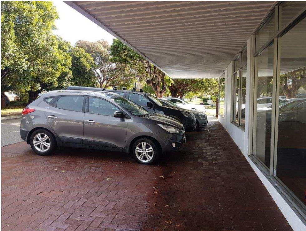
Figure 5 - Finding 4.3 – Obstructed Footpath
