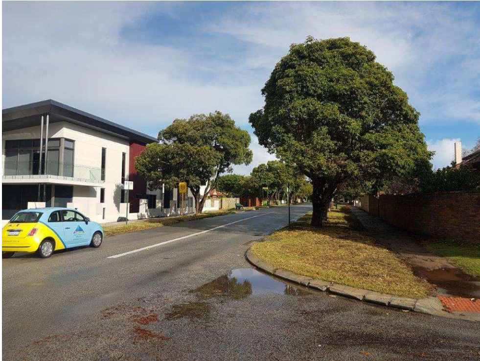
Figure 3 - Finding 4.1 – Sight Distance Obstruction
