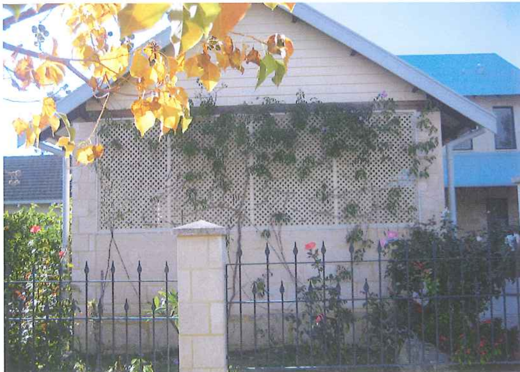
2. Photo above, showing solid limestone wall and lattice enclosing the front (south) of the carport
