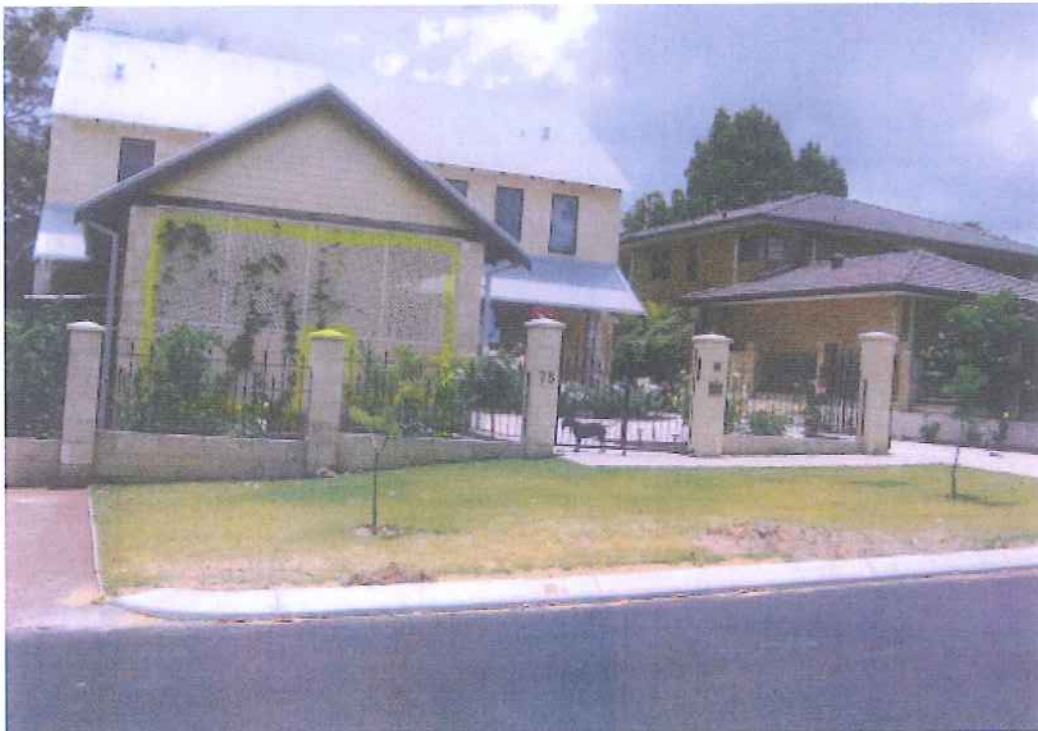
1. Photo above, showing enclosure to the front (south) of the carport, when viewed from street
