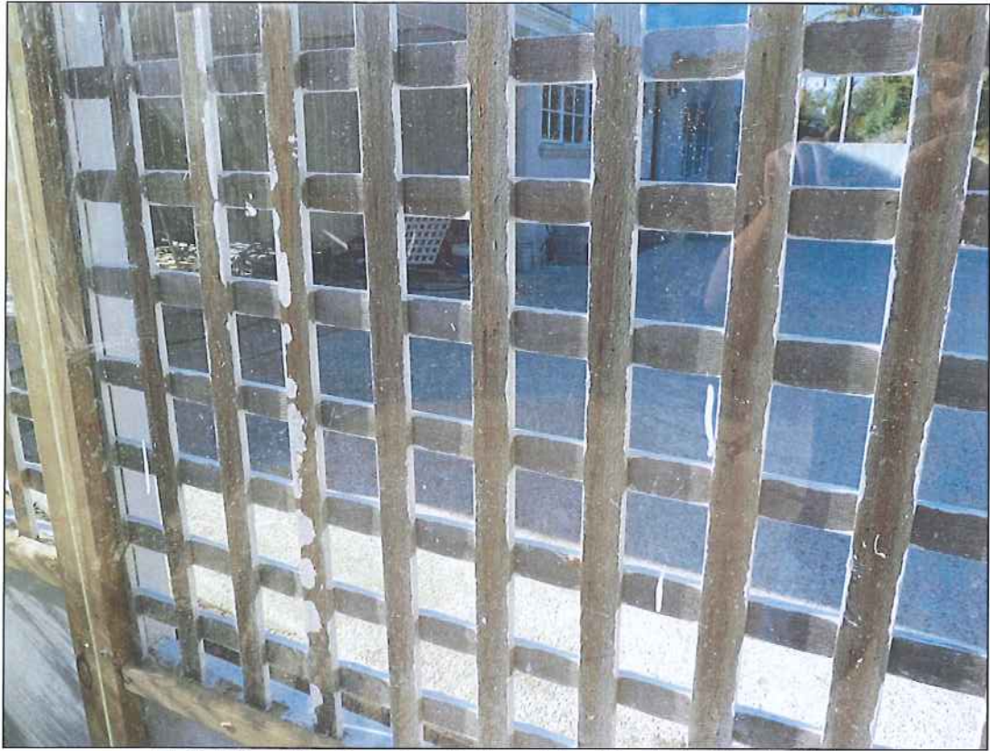
Unfinished Surface (partially painted & clad with plastic)
