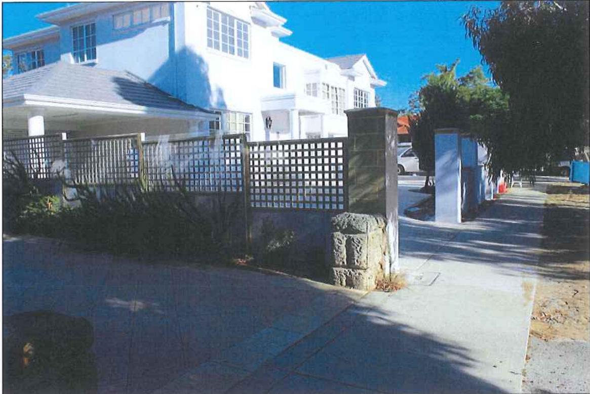
Side Dividing Fence between Nos. 97-101 Tyrell Street, Nedlands
