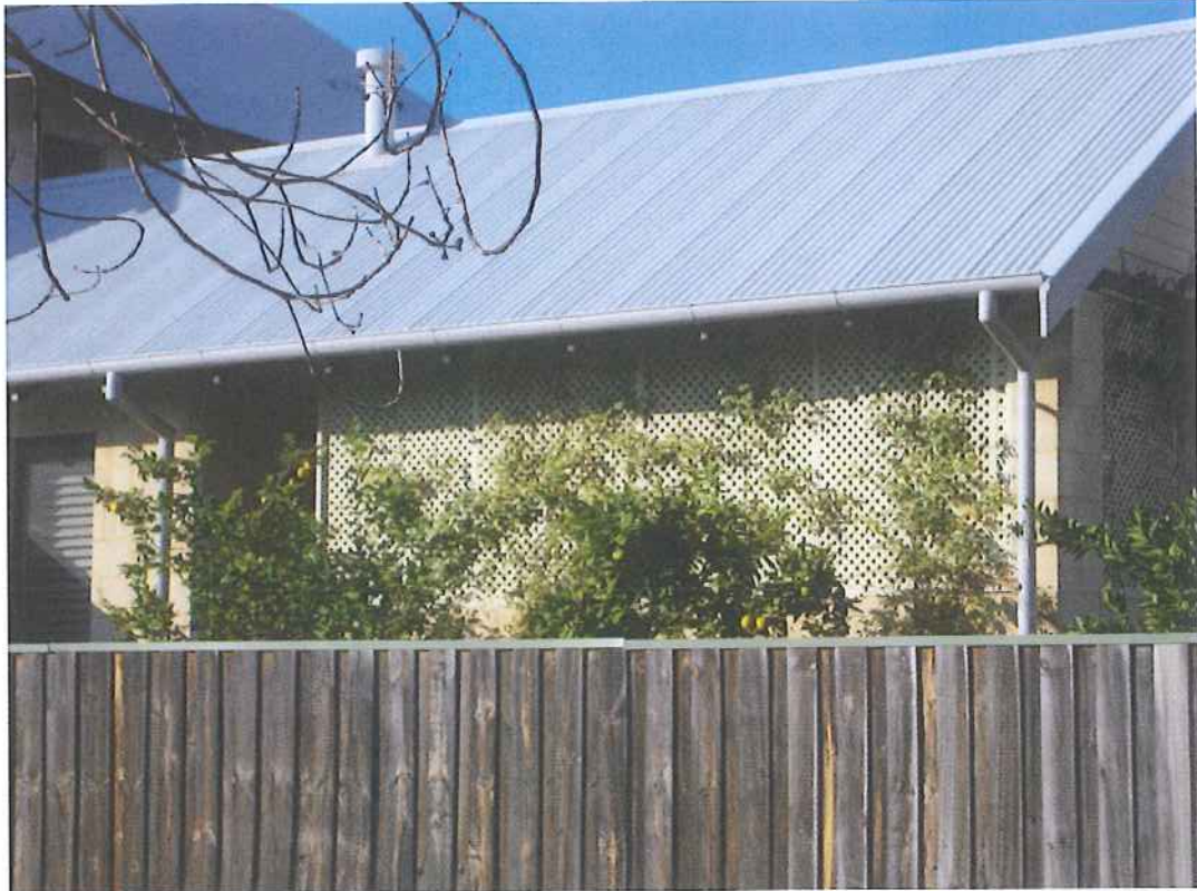
3. Photo above, showing enclosure to the side (west) of the carport
