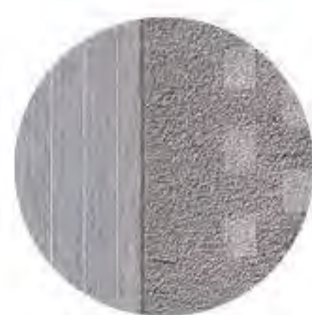
CONCRETE WALL WITH PATTERN
