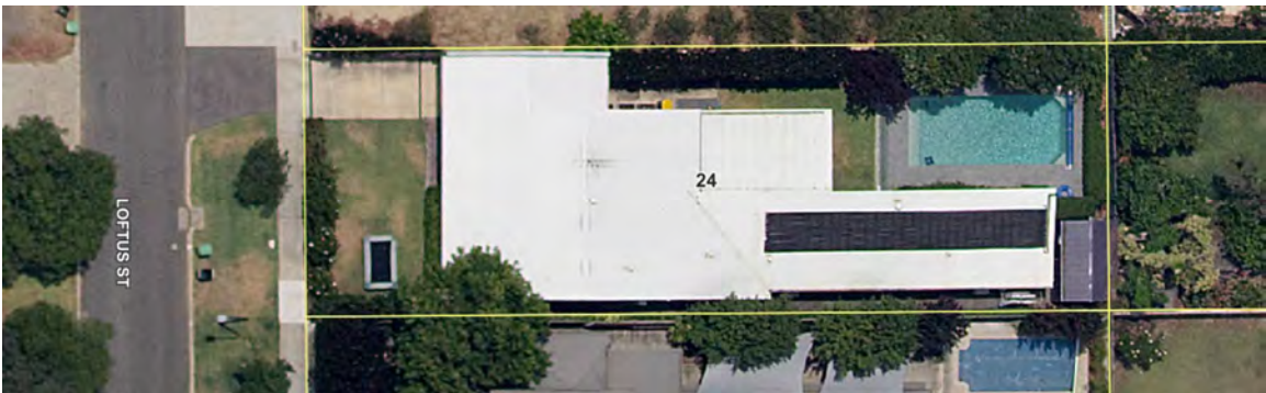
FIG 7. ARIAL PIC OF 24 LOFTUS STREET SHOWING THE EXTENSION THAT EXTENDS WELL OVER ITS BACK SETBACK BOUNDARY.
