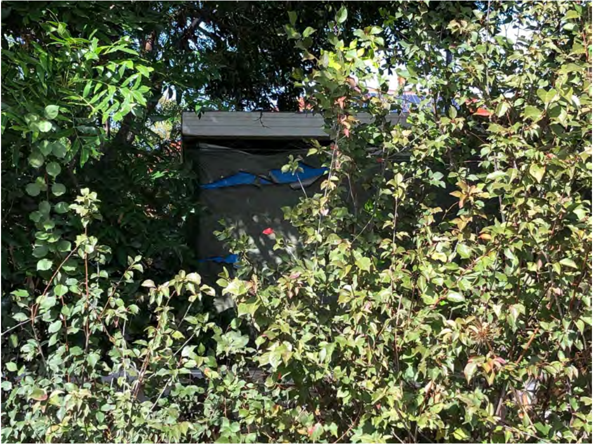
FIGURE 3. SHOWING AD-HOC STRUCTURE ALONG THE SOUTHERN BOUNDARY FACING CLI-ENTS PROPERTY THROUGH THE THICKET. THIS PROVIDES UNAPPEALING VISUAL IMPACT UPON CLI-ENTS RESIDENCE.
