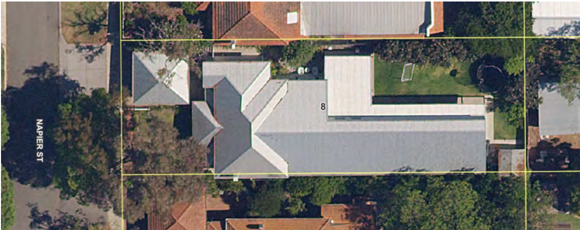
FIG 6. ARIAL PIC OF 8 NAPIER STREET SHOWING THE EXTENSION THAT EXTENDS WELL OVER ITS BACK SETBACK BOUNDARY.
