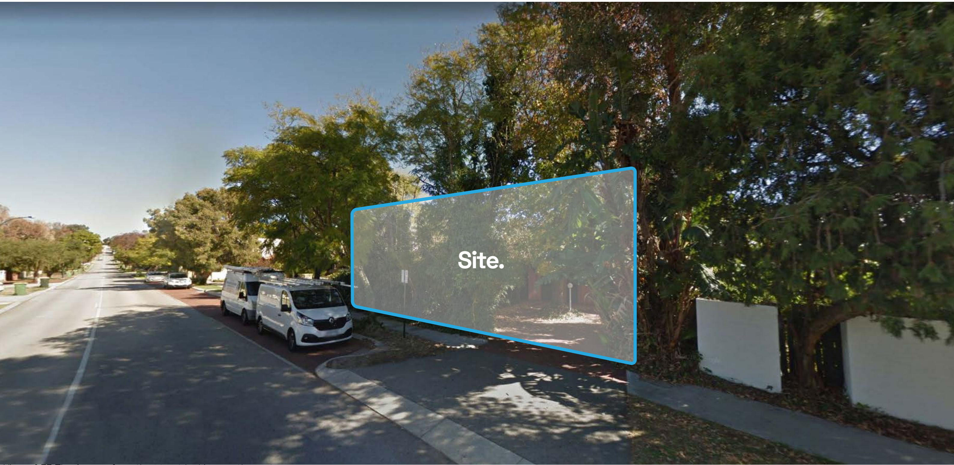
View of 35 The Avenue from the street looking south-west.
