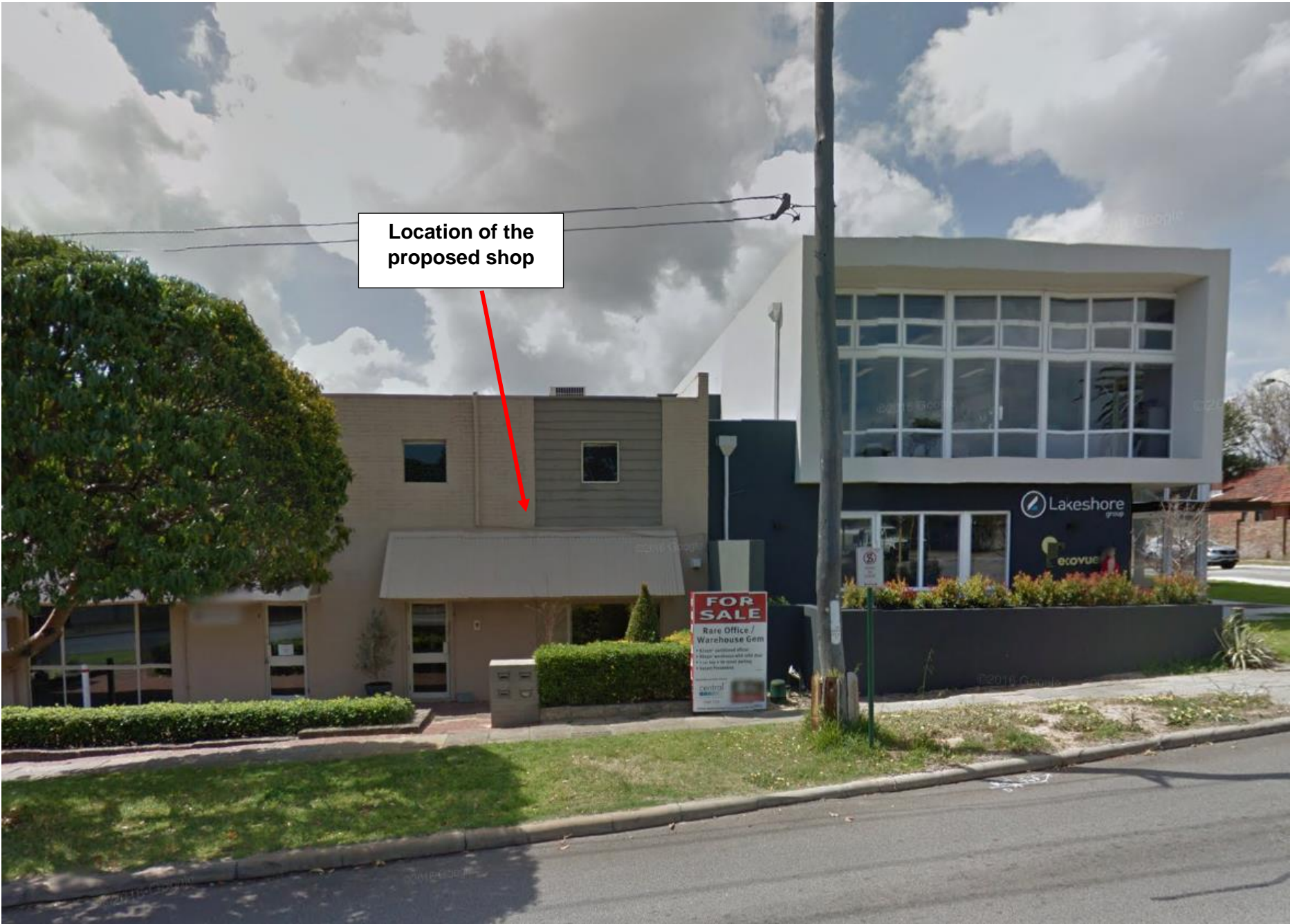
PD29.16 - Attachment 4 Photograph of 2A Loch Street
