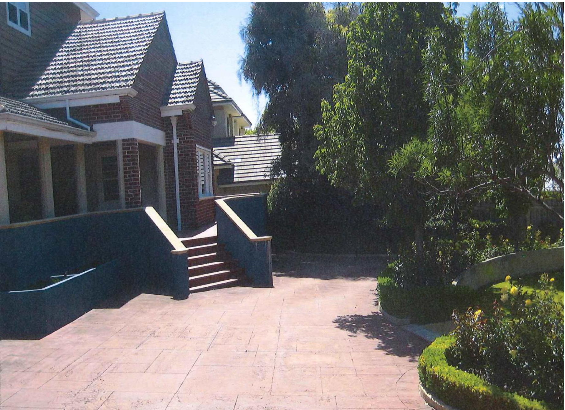
PD28.16 - Attachment 4 Photograph of 3 Bellevue Avenue taken from the air conditioning unit's location
