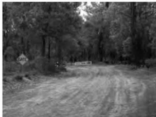
Figure 22: Emergency access ways may be used to link up with roads to allow alternative access during emergencies
