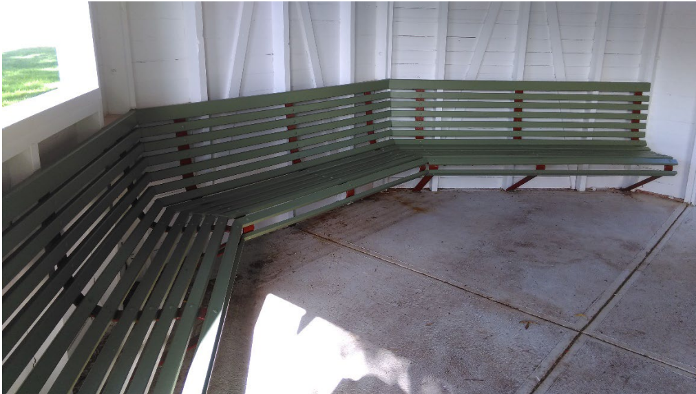
Figure 1: Internal refurbishment - April 2018
