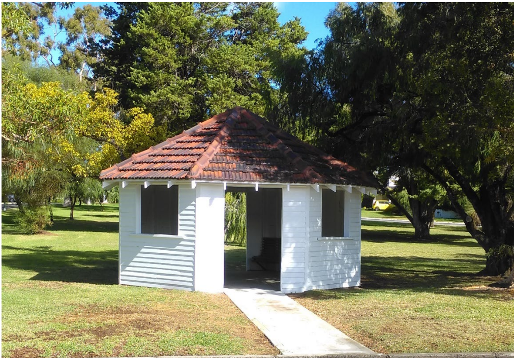
Figure 2: External refurbishment - April 2018
