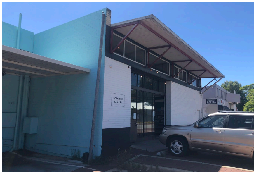
Figure 3 - No 29 Carrington Street / 27 Carrington Street, Nedlands
