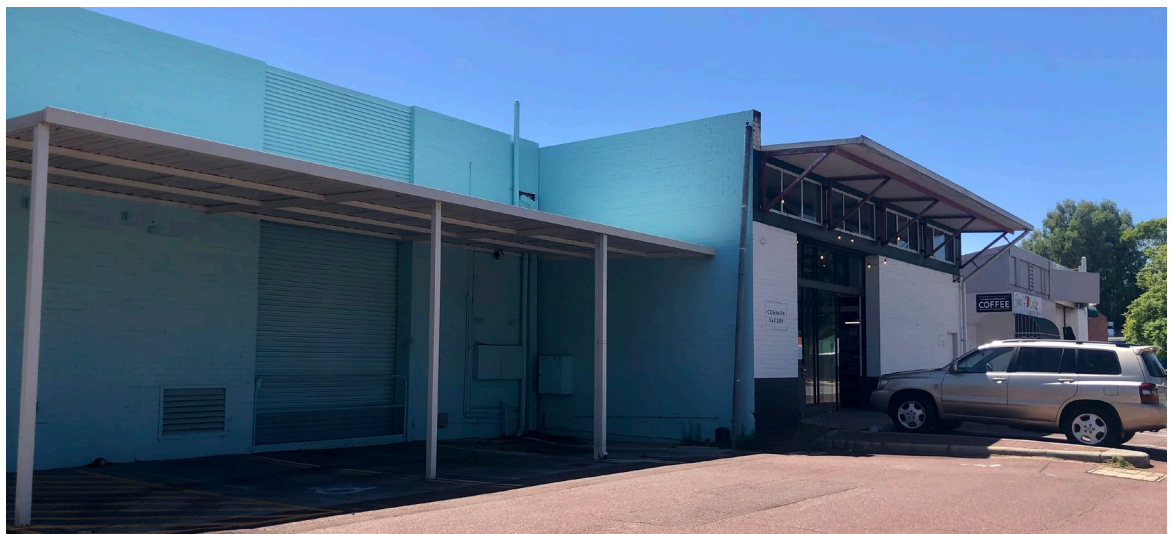
Figure 2 - No 29 Carrington Street / 27 Carrington Street, Nedlands
