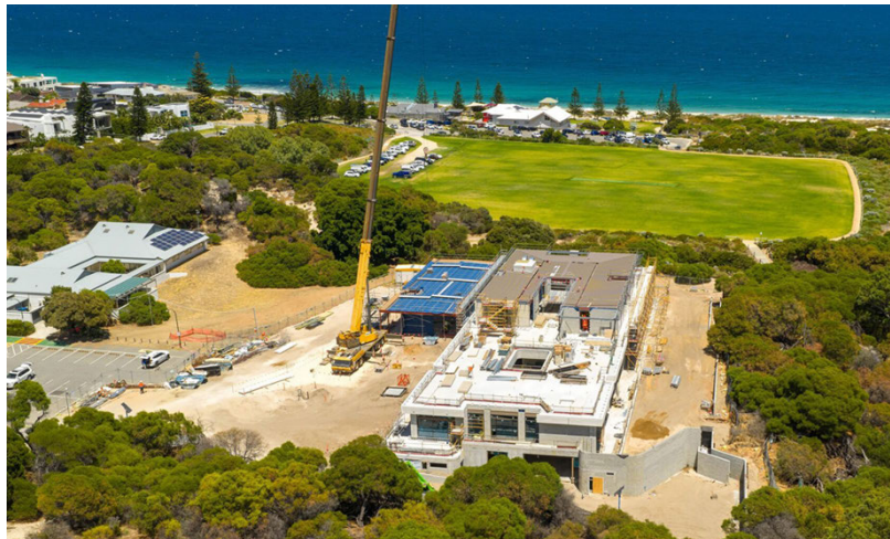
Figure 1. Hospice Development under construction (circa January 2026)
