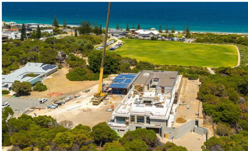
Figure 1. Hospice Development under construction (circa January 2026)
