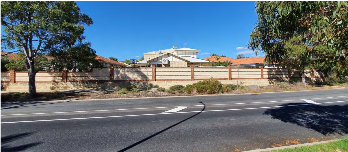
Photograph 5: Interface with existing properties (eastern side of street).
