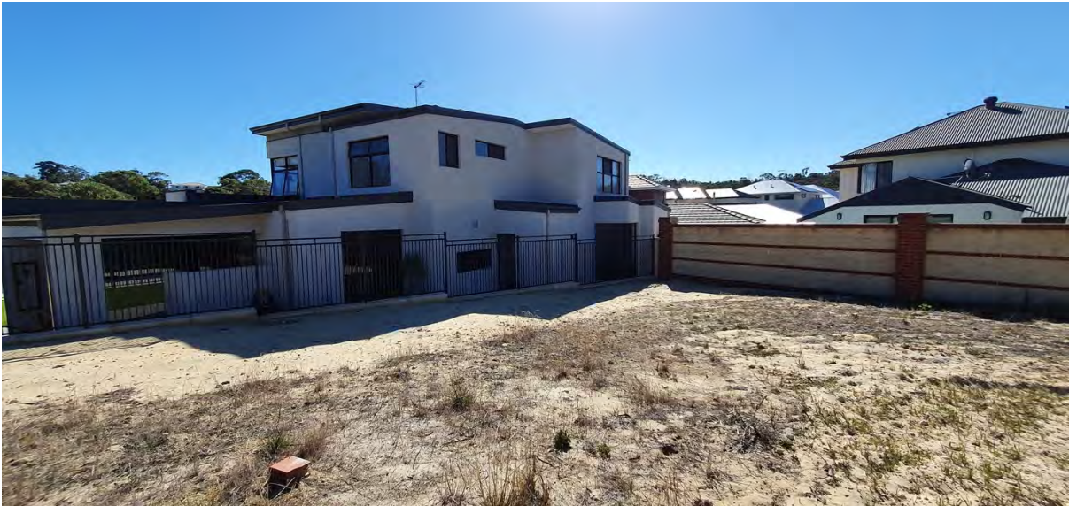
Photograph 7: Interface with existing properties (western boundary).
