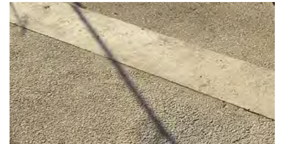
Insitu Concrete with Stone Inlay
